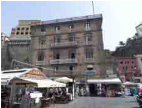
Fig. 1 – Marina Piccola Port area.
