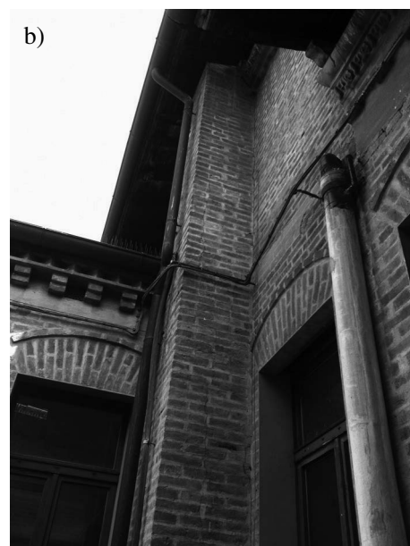
Fig. 21. A very large crack between two masonry walls (a) and a vertical crack between the chimney and the façade (b) of the primary school “Battisti”.
