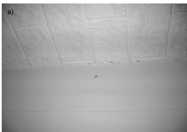
Fig. 25. Wall-floor cracks (a) and small vertical damage between orthogonal walls (b). Fessure parete-soffitto (a) e leggero danneggiamento tra pareti ortogonali (b).
