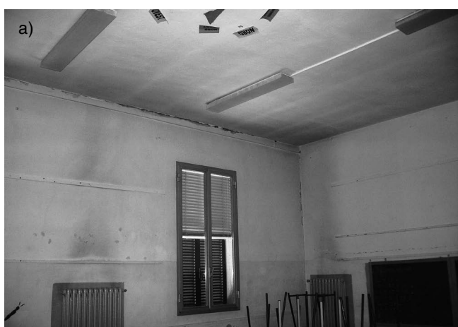
Fig. 13. Masonry structural unit of the school building "Menotti": wall-floor horizontal crack (a) and diagonal cracks into wall and floor (b).
