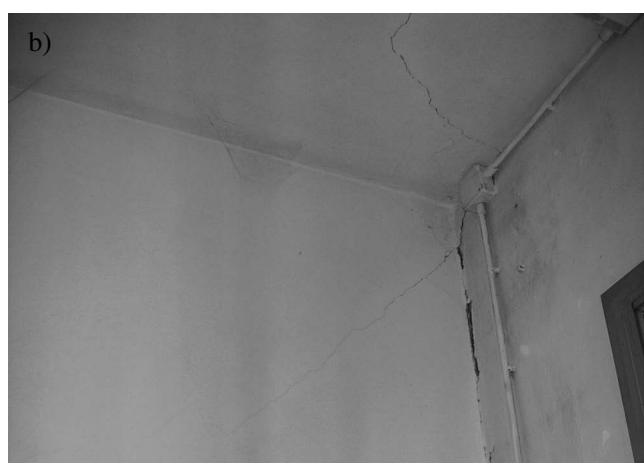
Fig. 13. Masonry structural unit of the school building "Menotti": wall-floor horizontal crack (a) and diagonal cracks into wall and floor (b).
