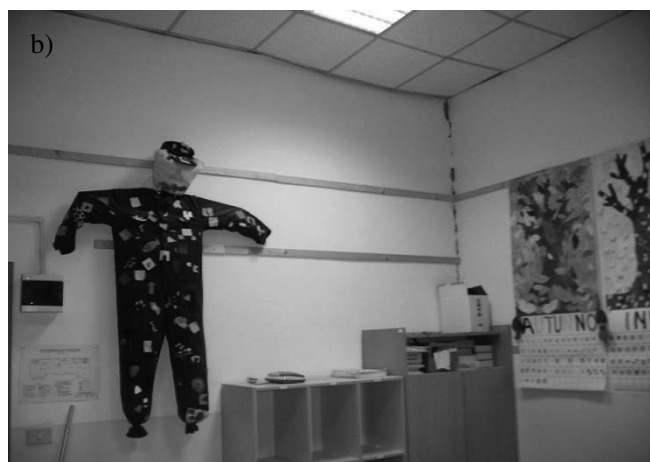
Fig. 2. Failure of ceiling panels (a) and vertical crack between masonry wall and internal one (b). Crollo di pannelli del controsoffitto (a) e fessure verticali tra parete in muratura e divisorio interno (b).
