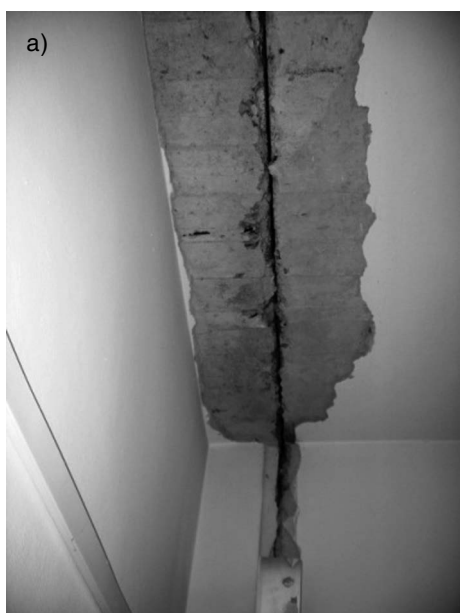
Fig. 5. Vertical crack corresponding to the joint zone (a) and a slight foundation subsidence at the building base (b). Fessure verticali in corrispondenza del giunto (a) e leggero cedimento della fondazione (b).
