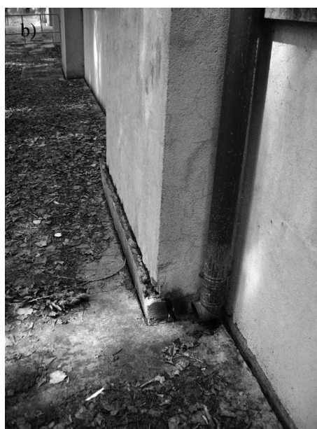
Fig. 5. Vertical crack corresponding to the joint zone (a) and a slight foundation subsidence at the building base (b). Fessure verticali in corrispondenza del giunto (a) e leggero cedimento della fondazione (b).
