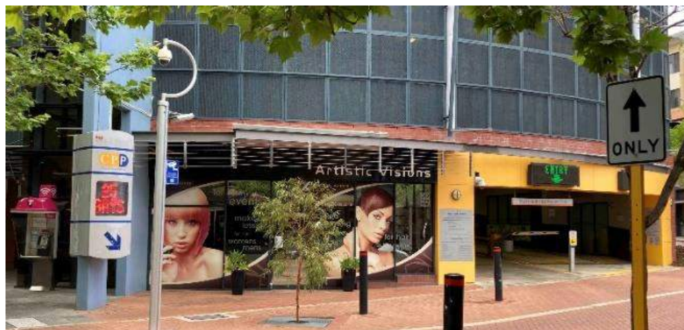
Figure 7. Parking structure. Copyright: Liang Wen.
