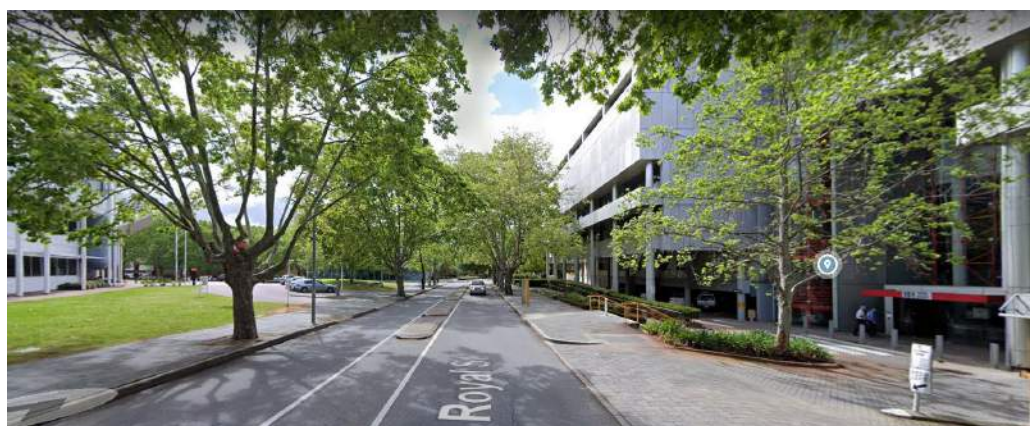
Figure 11. Ground floor of the Central TAFE College (on the left side) and Department of Education (on the right side) used for parking. Source: Google Streetview.
