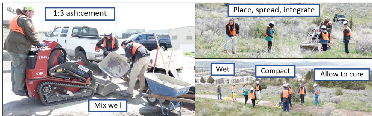
Figure 3.3: Process for applying Mt. Mazama ash treatment to trail surface.
