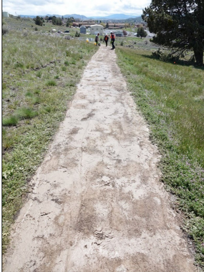
Figure 3.4: Completed trail surface.
