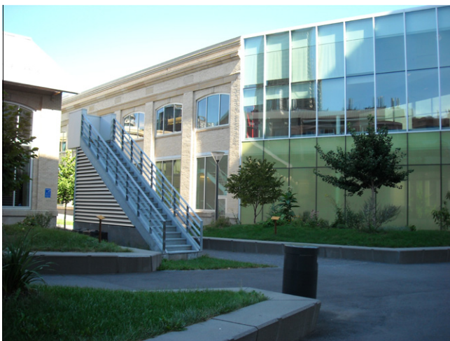
Fig. 2. (File number 2234), courtyard of the Complexe des Science, Université du Québec à Montréal. The design highlights links between the sense of community and natural environment.
