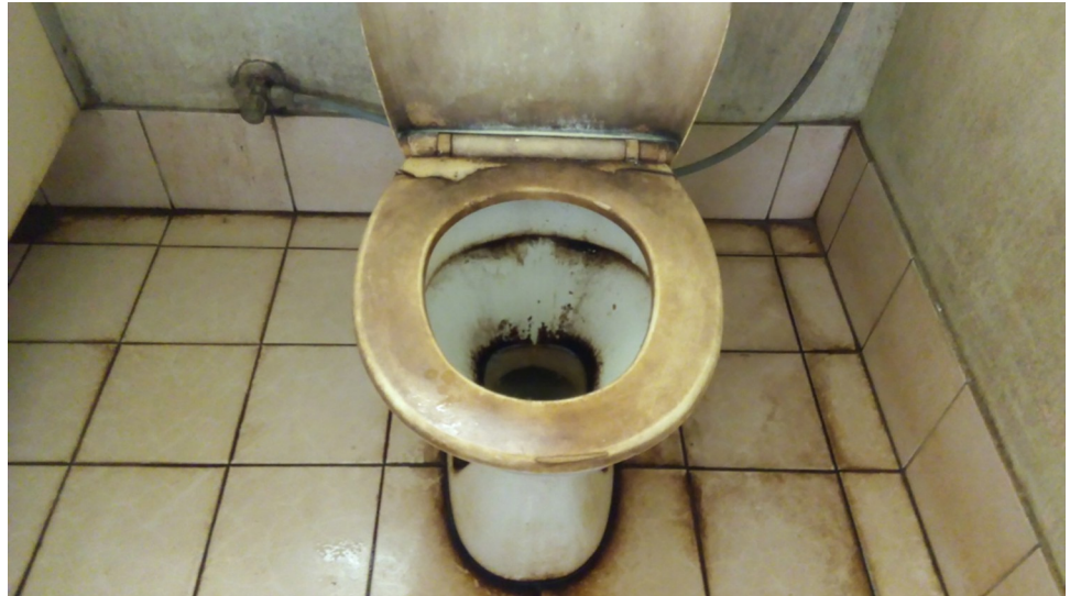
Fig 3. CP5 (A dirty toilet).
