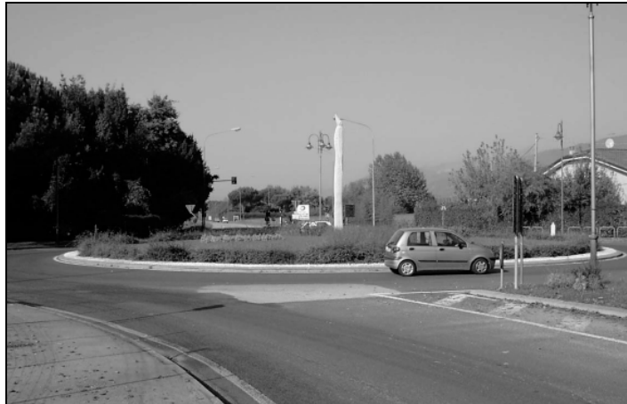
Figure 6: The Folon's obelisk in Pietrasanta (Lucca, Italy) is an example of the central island "slender" development.
