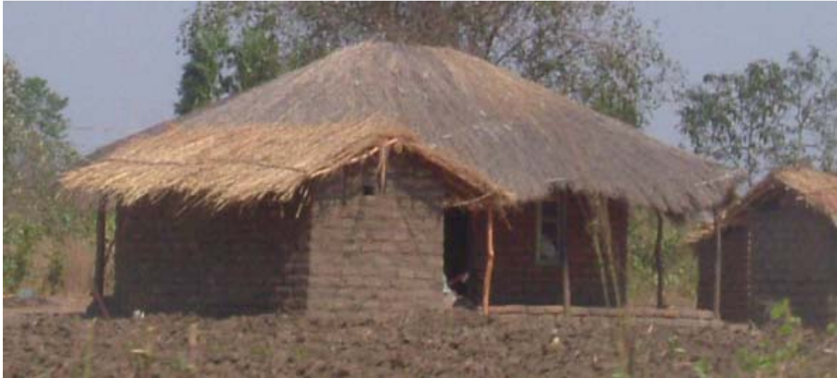
Fig. 1: A traditional building in sub-Saharan Africa
