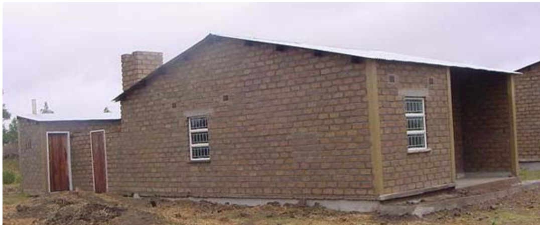
Fig. 15: Stabilised Soil Block Teacher's House at Namadidi Primary School in Phalombe
