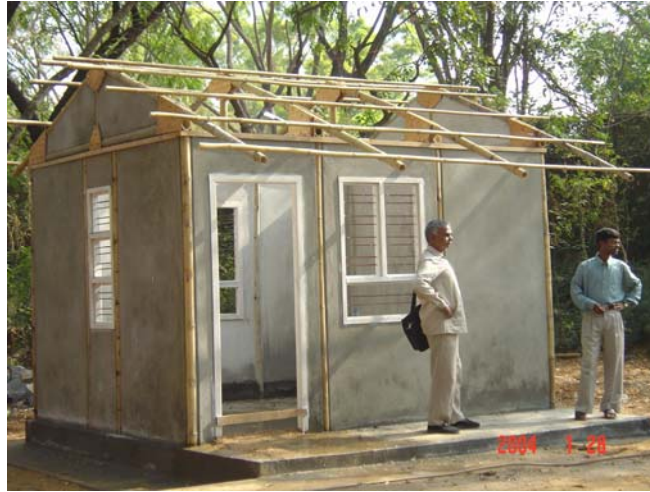
Fig. 17: Demonstration of a bamboo framework for housing
