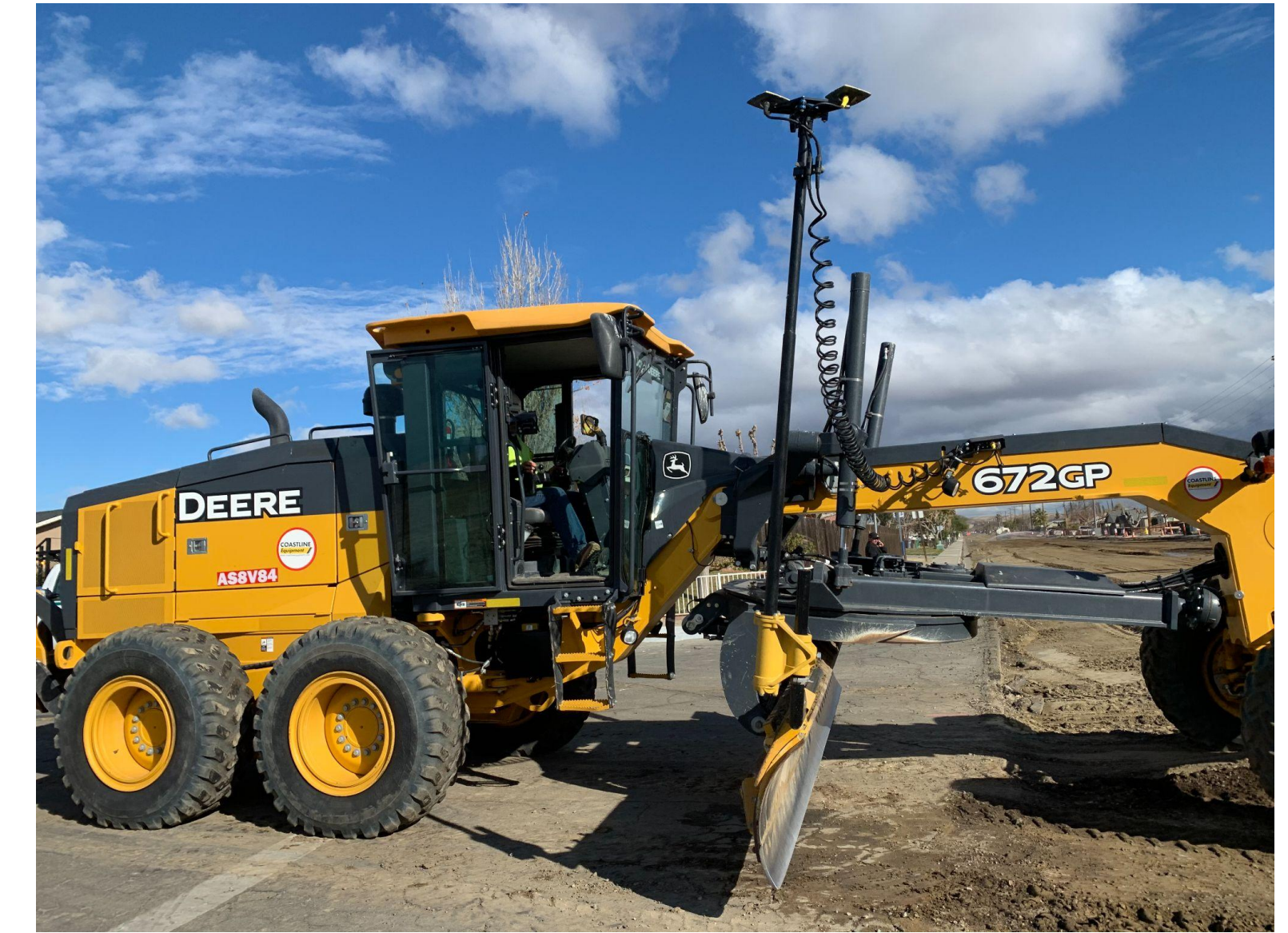
Traditional Motor Grader with GPS Cabling & Mast
