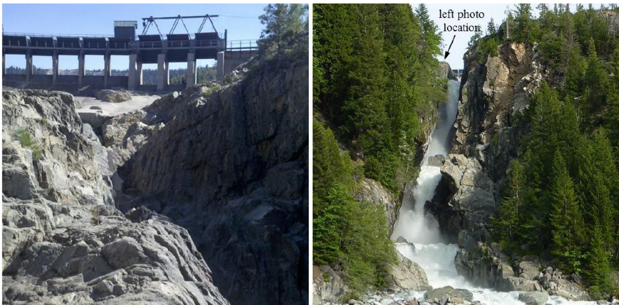
Figure 1. Upper reach of eroded slot canyon viewed from middle of spillway (left) and lower reach of slot canyon viewed from below with alluvial fan of scoured material in the foreground (right).
