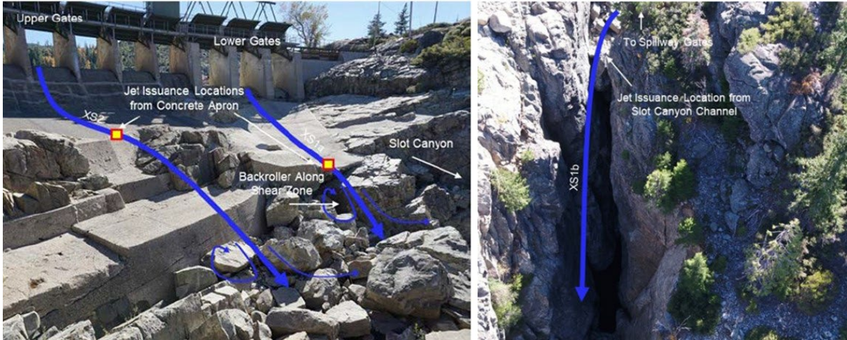
Figure 3. Cross-sections XS 1a and XS 2 for jets emanating from the concrete apron from the lower and upper spillway gates, respectively (left) and XS 1b for jet emanating from the slot canyon channel.
