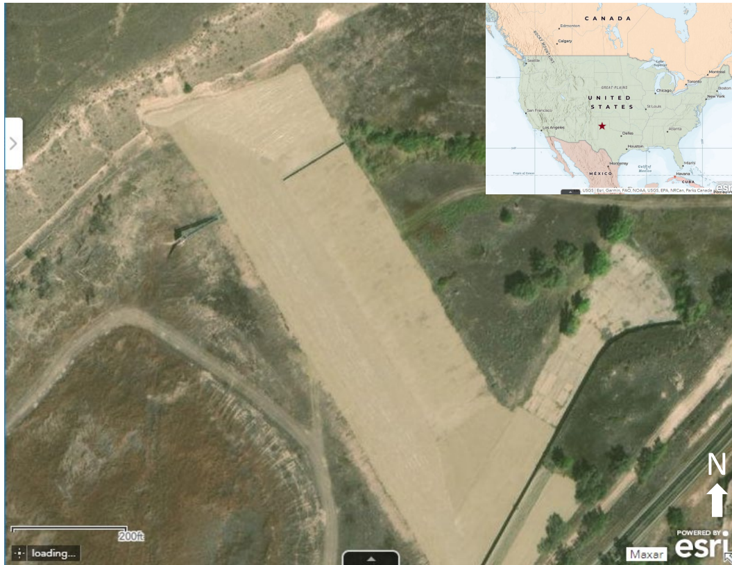
Figure 1: Umbarger Dam aerial photograph and location map (inset).
