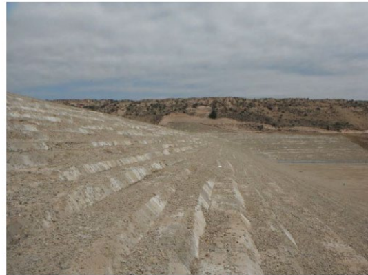
15. Downstream slope, looking left from near STA 7+50.
