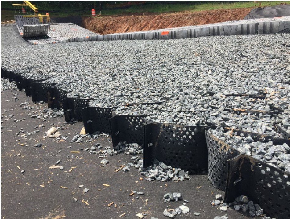
Figure 2. Geocell stabilized drainfill.
