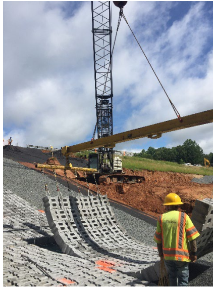
Figure 1. ACB installation.
