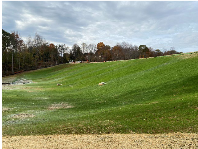
Figure 9. Finished embankment covered with topsoil and seed.
