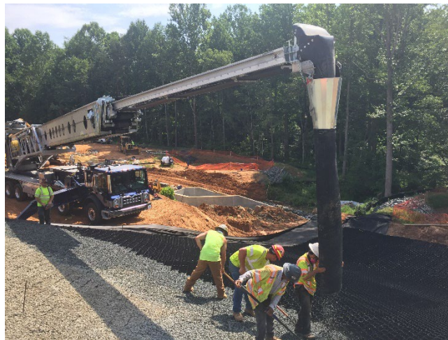
Figure 7. ACB drainfill placement.
