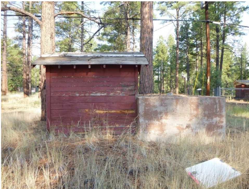
Figure 32. Exterior of Old Well House (16-71), view west.
