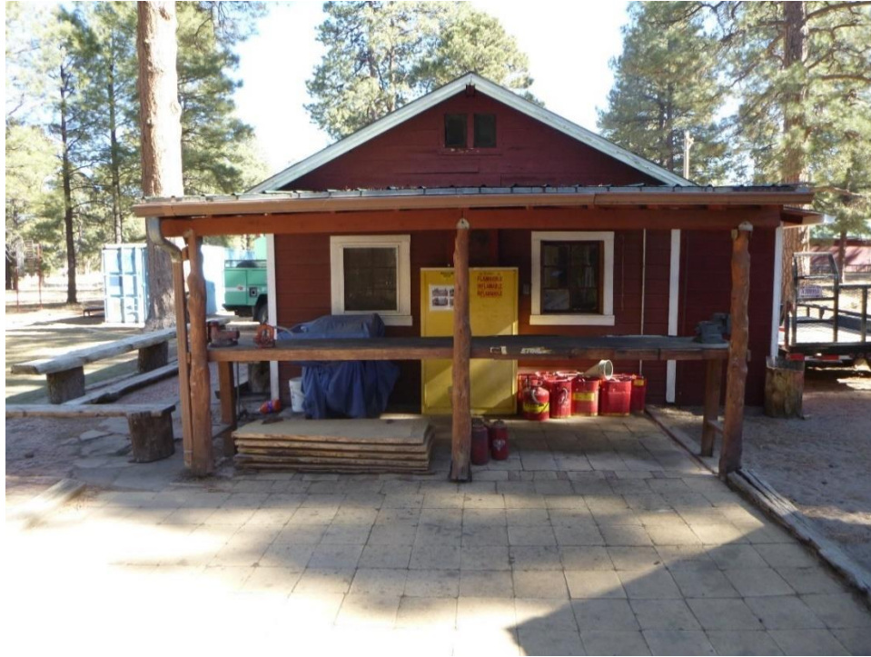
Figure C.67. Backside of Hotshot building (13-91), view north.
