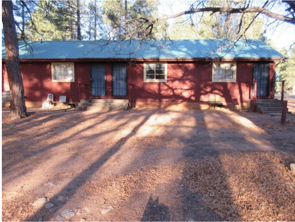
Figure C.21. East side of Engine Quarters (11-60), view west.
