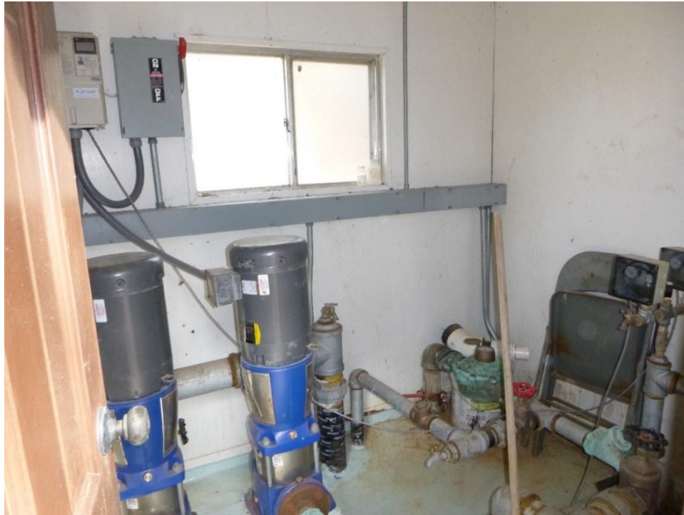
Figure 35. Interior of Chlorine/Pump House (12-17), view from doorway.
