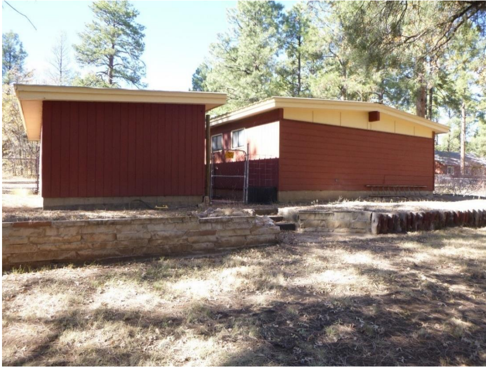
Figure 17. Ranger House exterior (11-40), view east.
