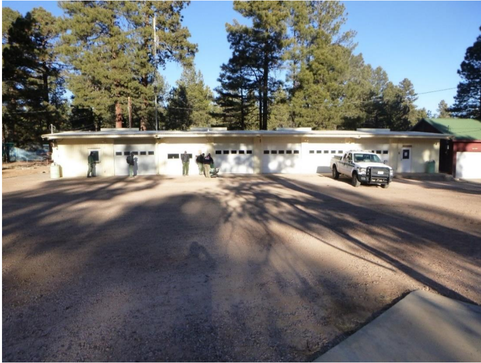
Figure 36. Shop exterior (13-84), view west.
