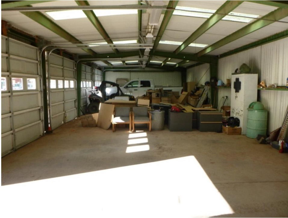
Figure 45. Interior of Garage 12 Bays building (13-91), view from center of building.
