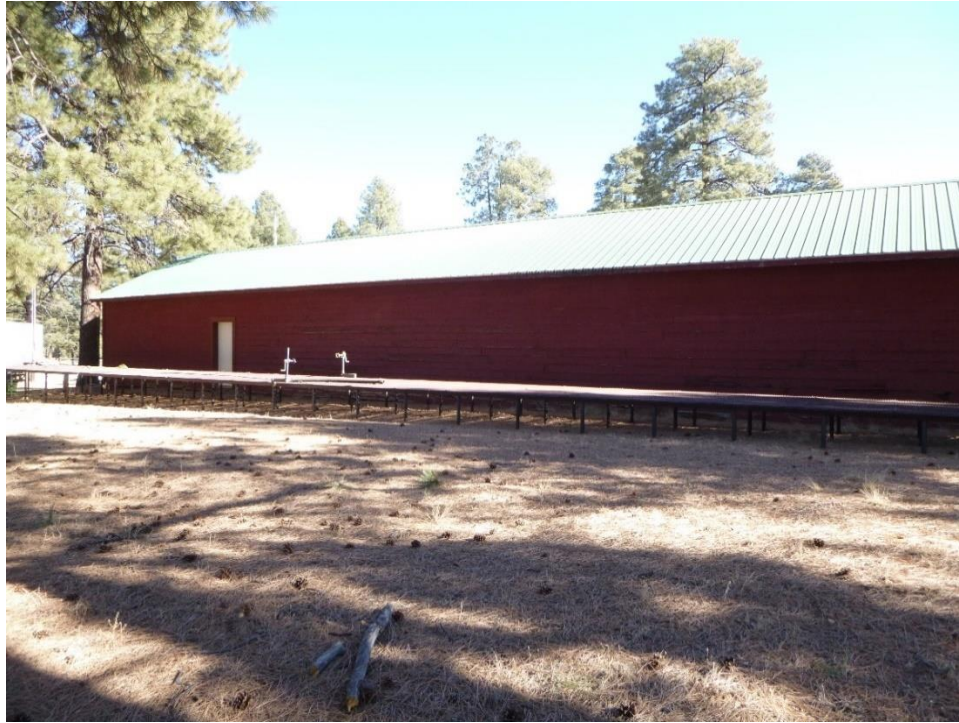
Figure C.61. Backside of the Fire Cache & Equip. Storage (13-30), view northwest.
