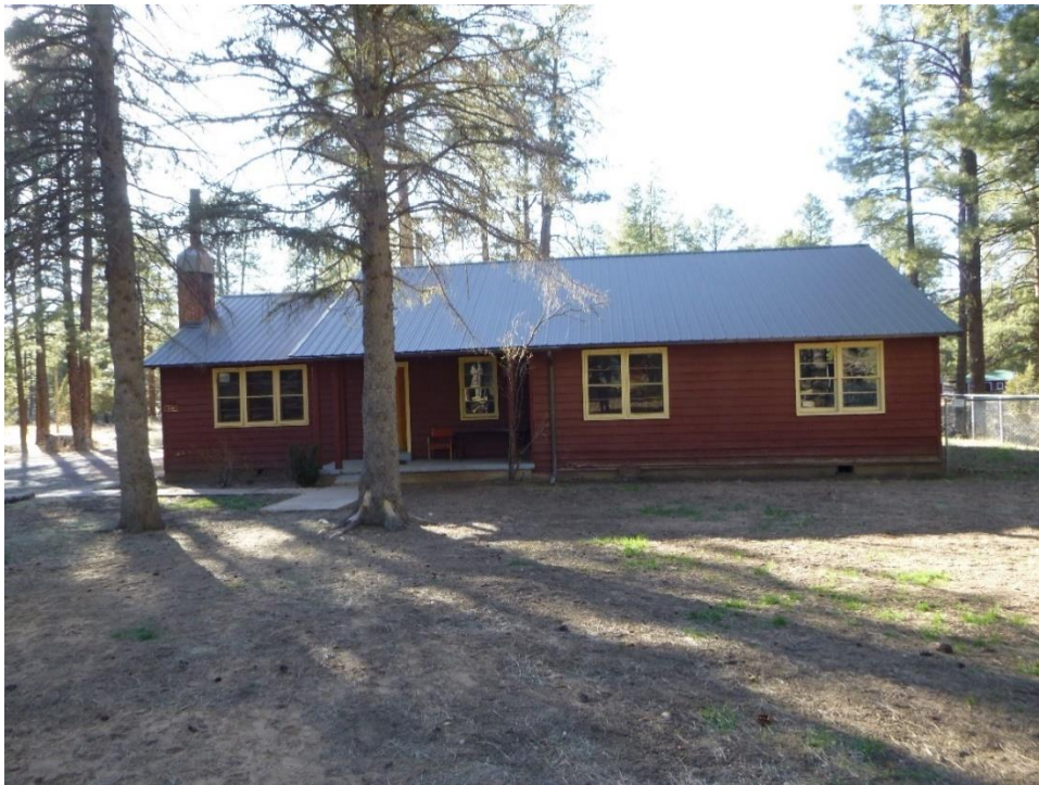
Figure 30. Weight Room building (11-54), view west.
