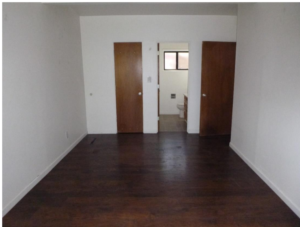
Figure C.14. Main bedroom with attached bath in Ranger House (11-40), view from north wall.
