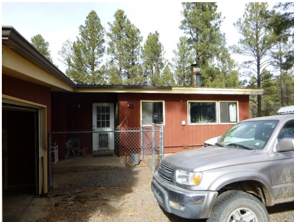
Figure C.29. Backdoor of Range House (11-38), view west.
