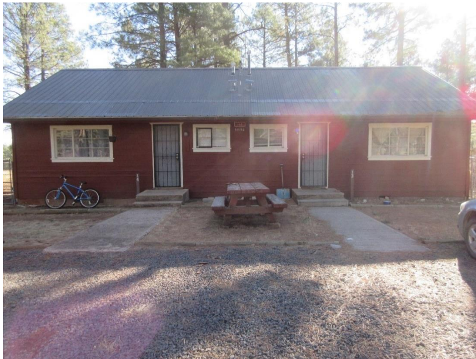
Figure 19. Old Duplex building (11-7), view east.
