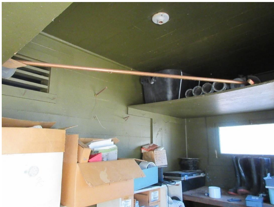
Figure C.6. Back storage room of Garage (13-67), view from garage area.
