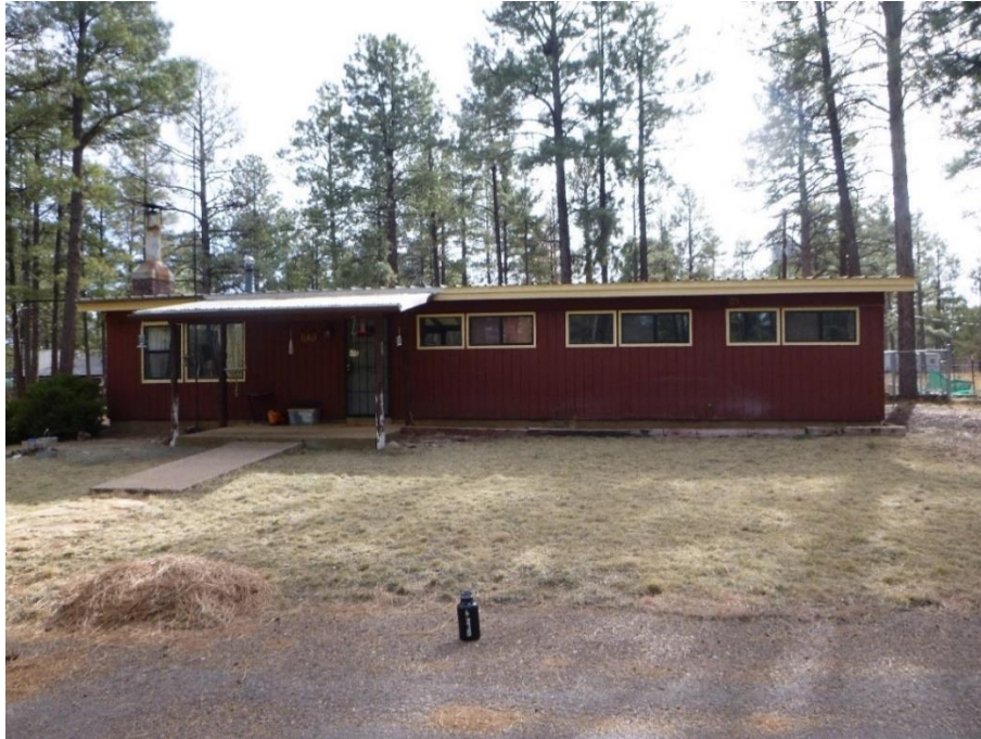
Figure 24. Range House exterior (11-38), view east.
