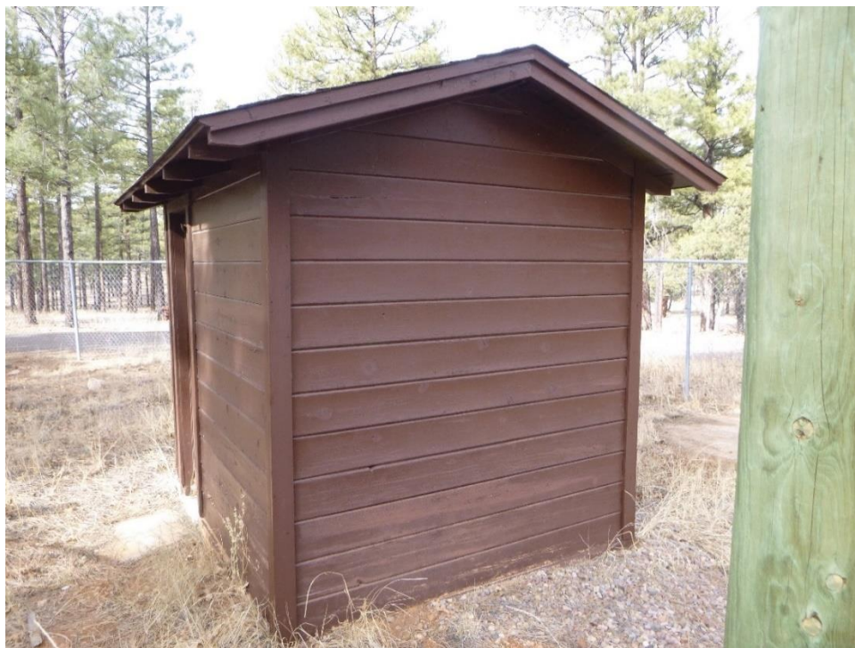
Figure C.50. Exterior of Chlorine/Pump House (12-17), view west.
