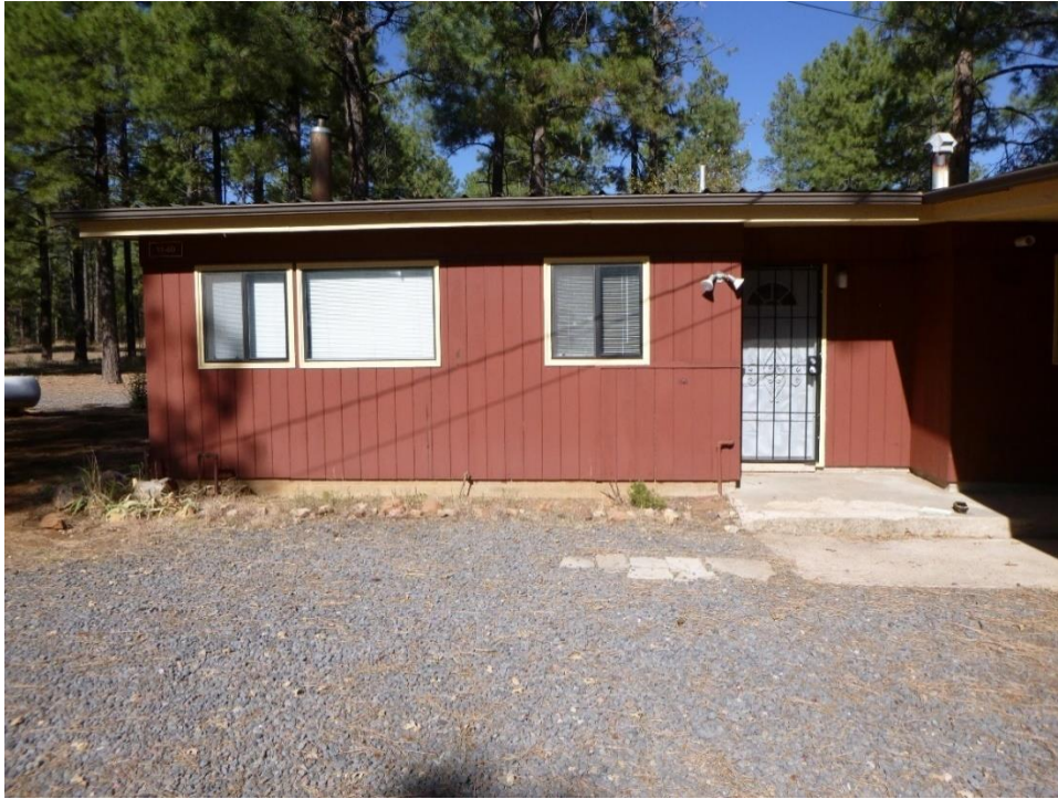
Figure 18. Ranger House exterior (11-40), view north.
