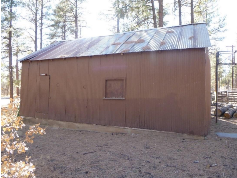
Figure 26. Exterior of Barn (13-69), view south.
