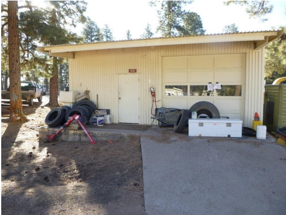
Figure 40. Paint and Gas building (13-94), view east.
