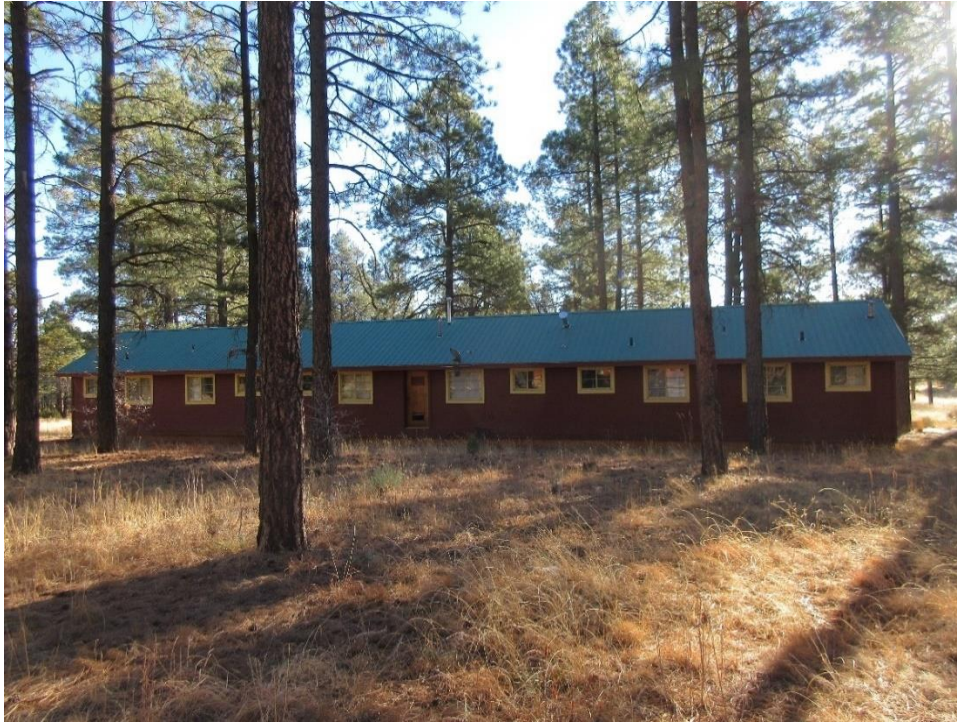
Figure 21. Engine Quarters building (11-60), view east.
