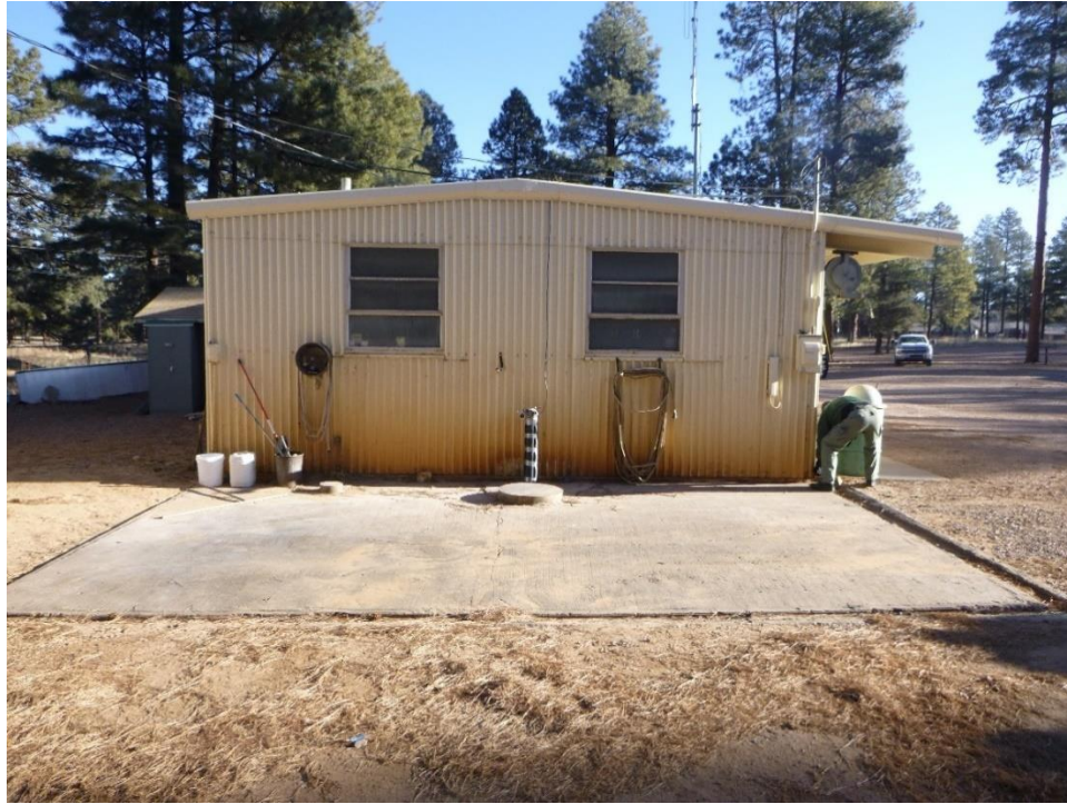
Figure C.52. South end of Shop (13-84) with truck wash area, view north.
