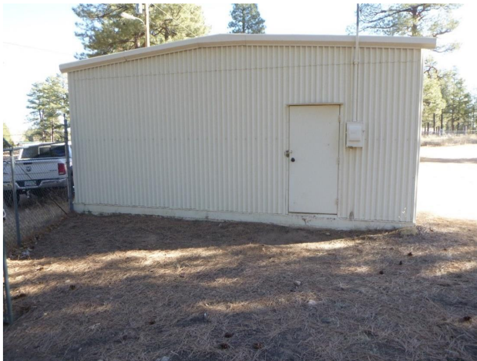
Figure C.64. South end of Garage 12 Bays (13-91), view north.
