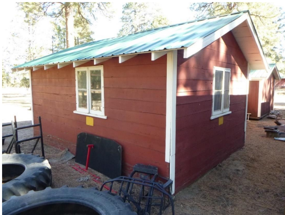
Figure C.70. South and west side of Hotshot Tool Shed, view northeast.
