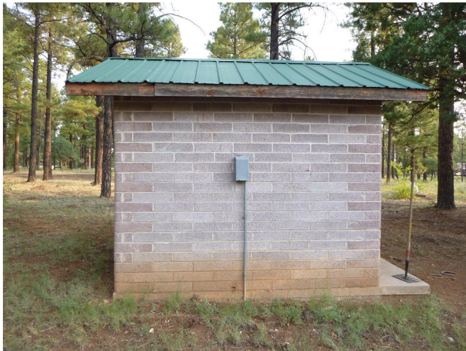
Figure C.26. South side of Radio building (15-93), view north.
