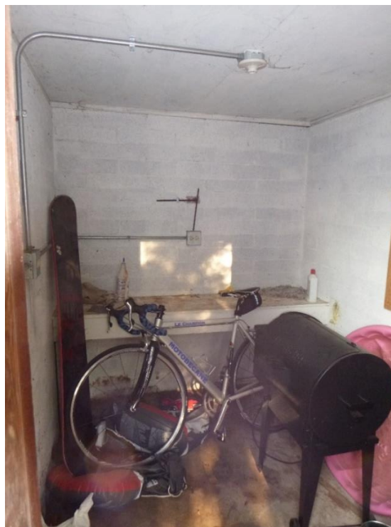
Figure C.27. Interior of Radio building (15-93), view from door.
