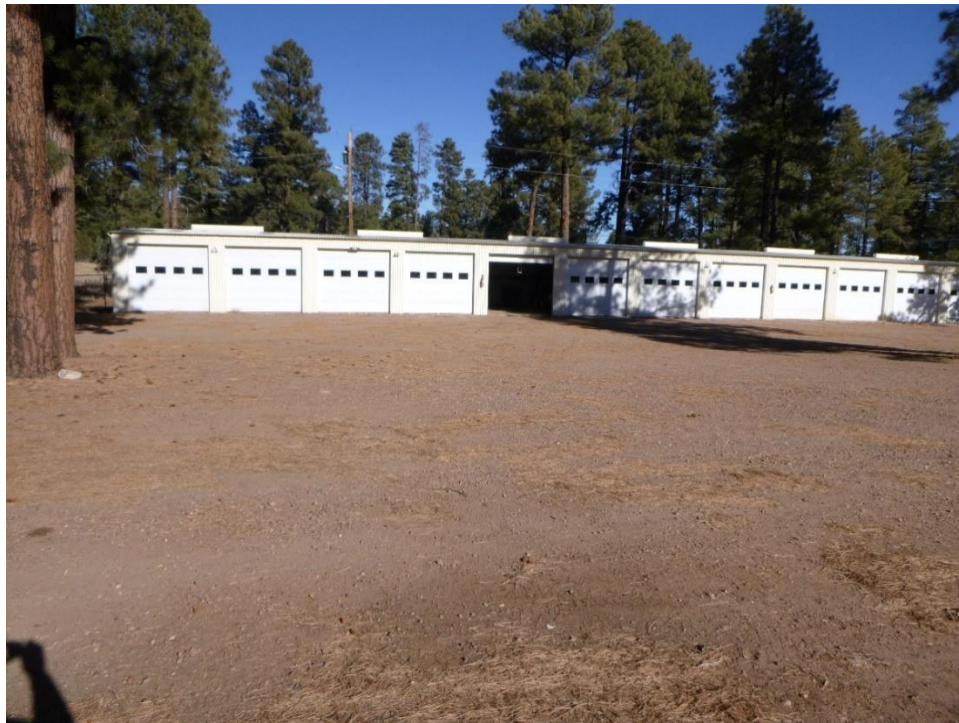
Figure 44. Garage 12 Bays (13-91), view west.
