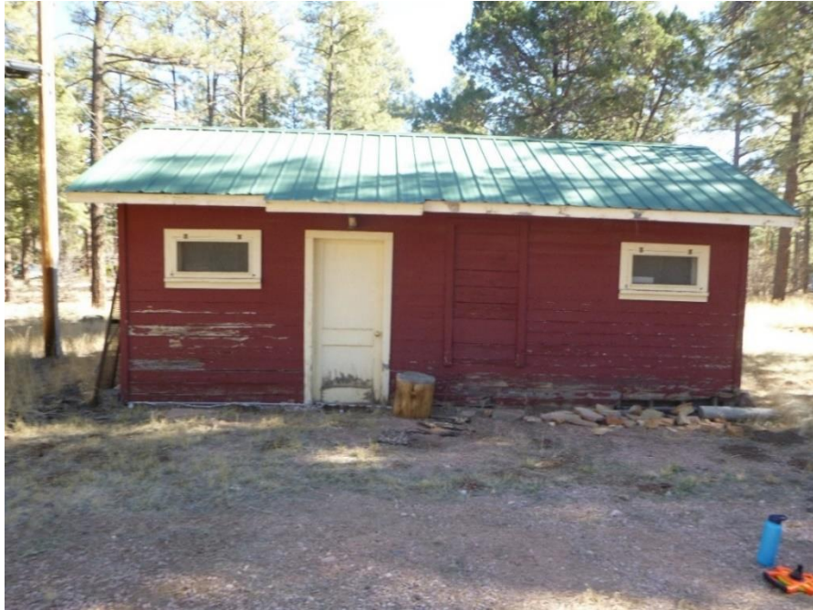
Figure 13. Garage building (13-67), view east.
