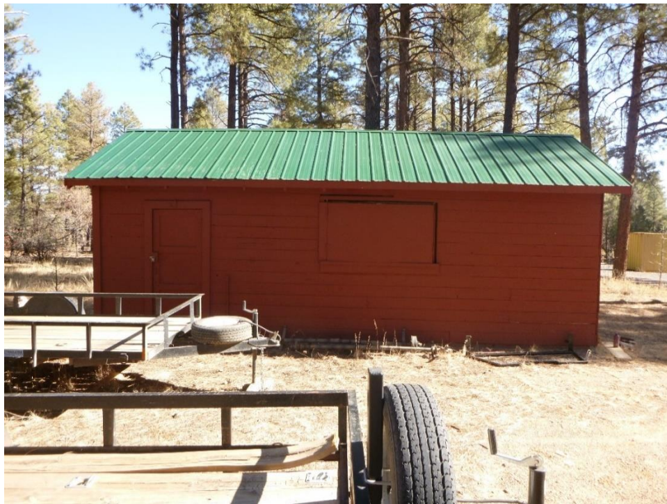
Figure C.8. West side of Garage, view east.
