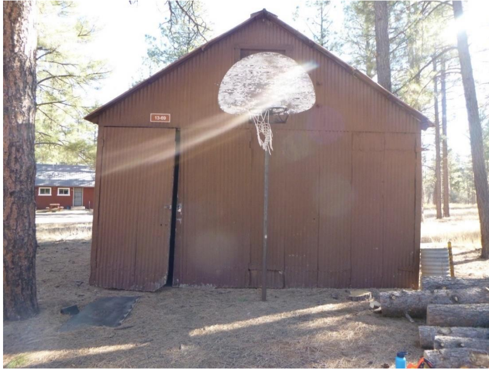
Figure C.34. Front of Barn (13-69), view east.
