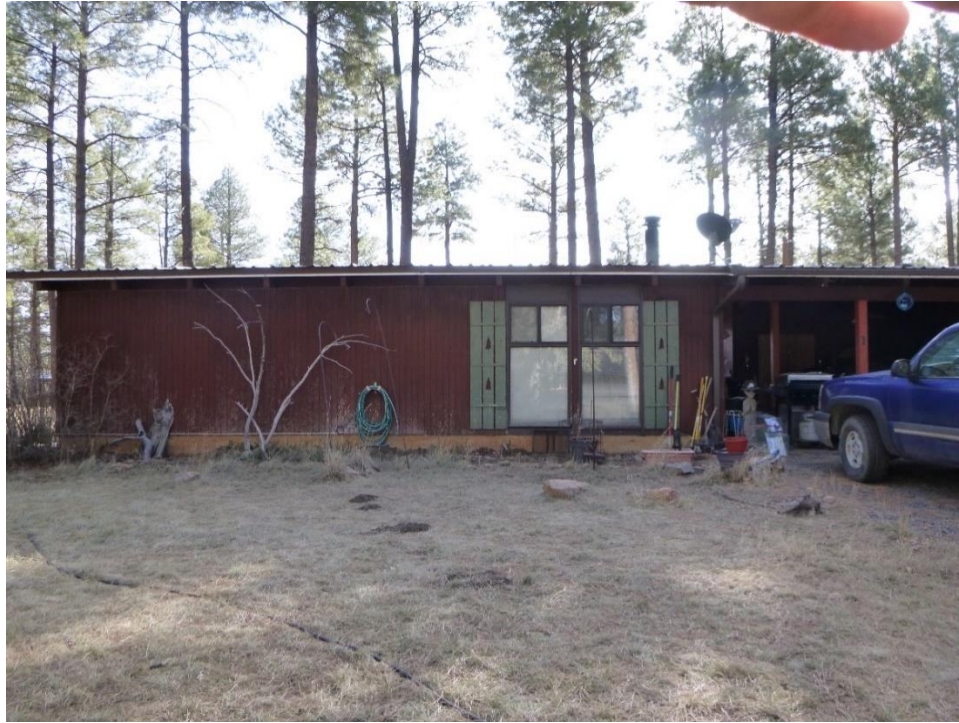
Figure C.37. North end of Duplex (11-85), view east.
