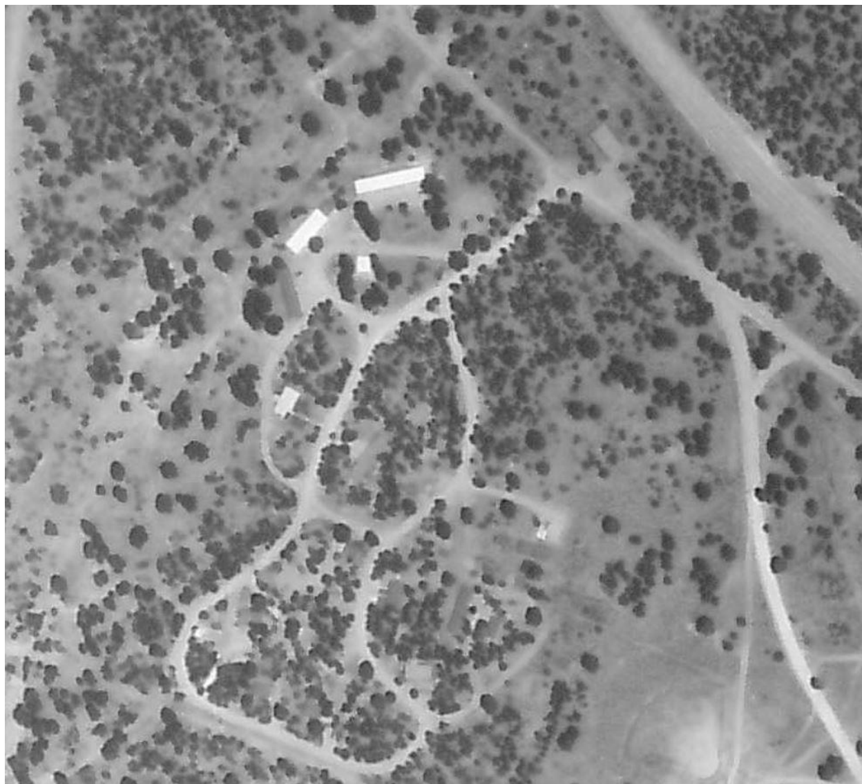
Figure A.9. ASNFs Black Mesa Ranger Station, 1968, aerial photograph of the Black Mesa Ranger Station.
