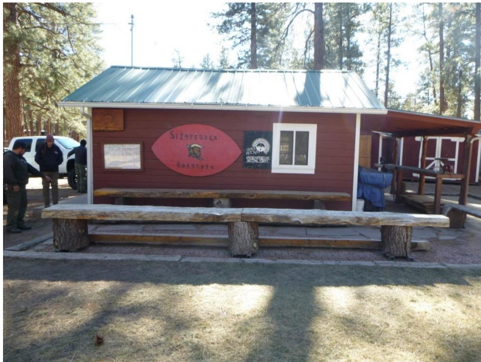
Figure C.68. West side of Hotshot building (13-91), view west.
