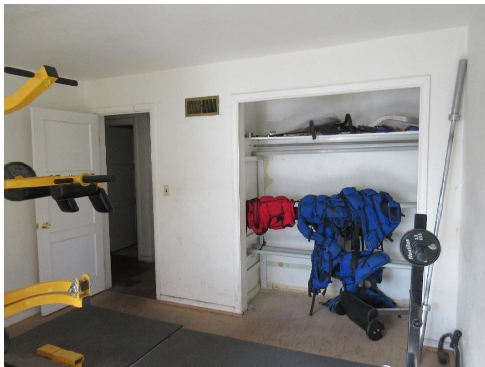
Figure C.44. Northeast bedroom in Weight Room (11-54).
