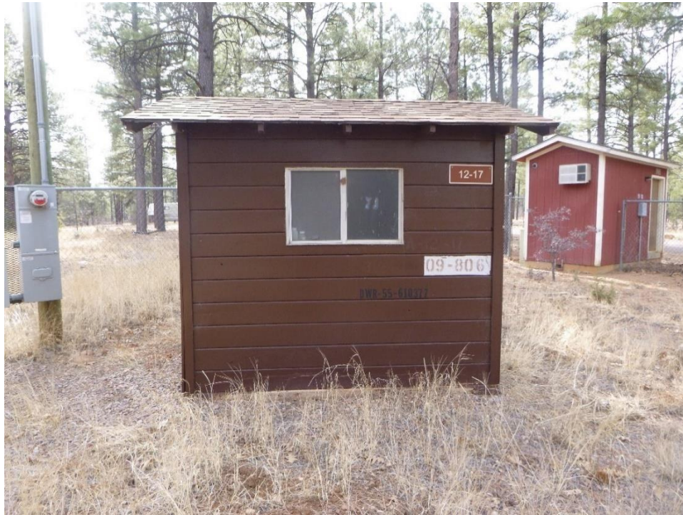
Figure 34. Chlorine/Pump House (12-17), view east.
