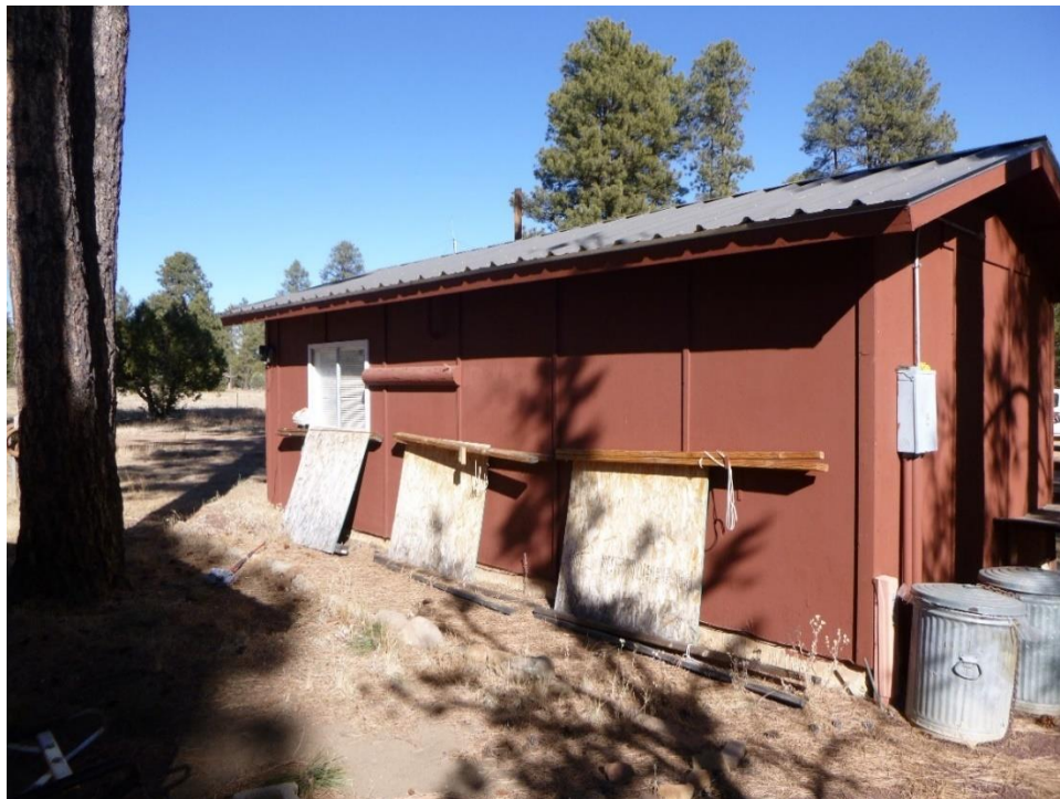
Figure C.3. Backside of Helibase (16-2), view northwest.
