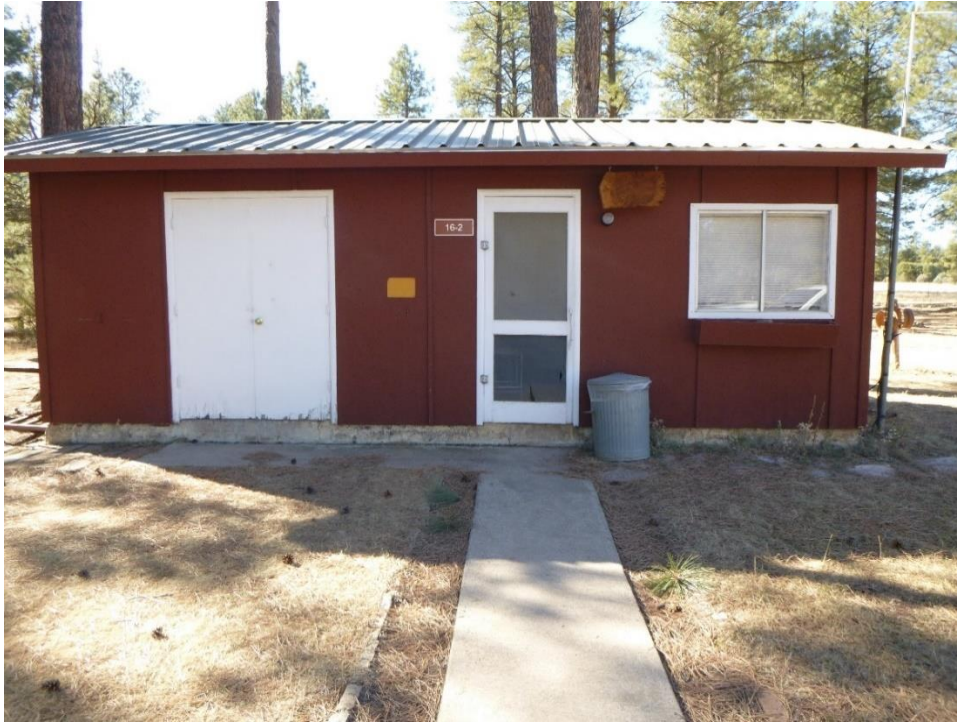
Figure 11. Helibase building (16-2), view south.
