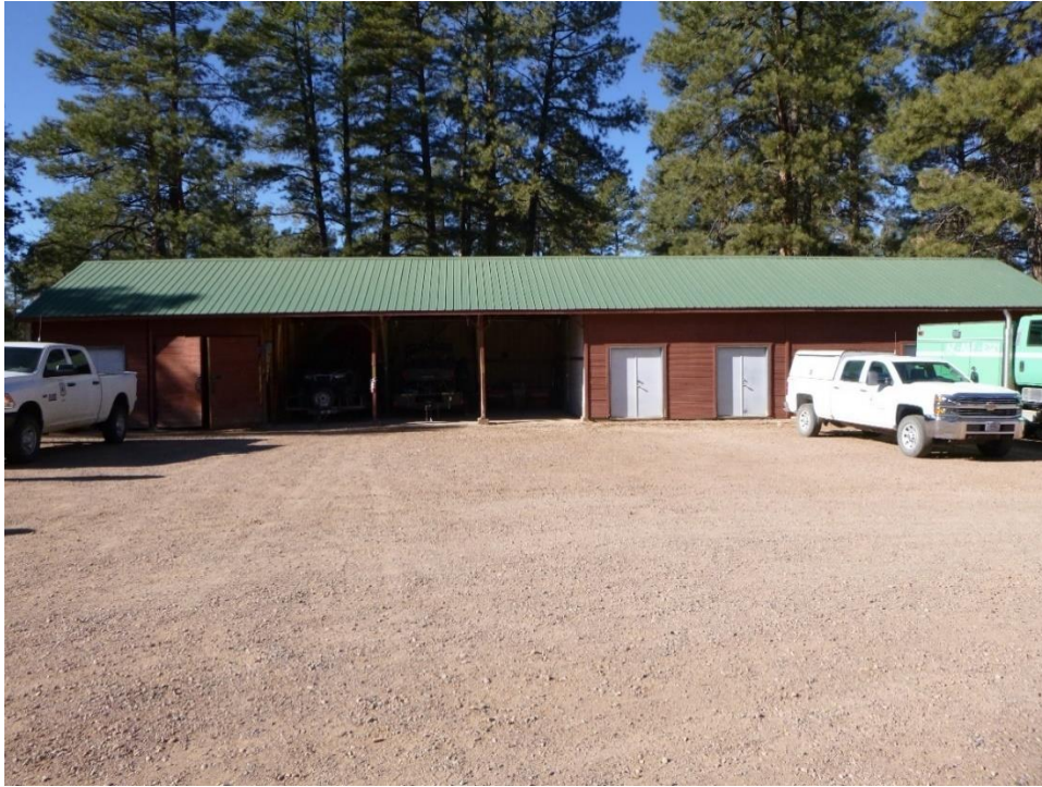
Figure 42. Fire Cache & Equipment Storage (13-30), view south.
