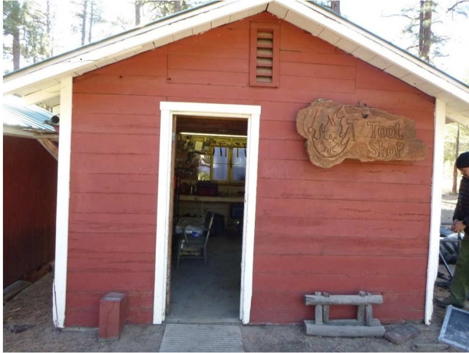
Figure 48. Hotshot Tool shed, view south.
