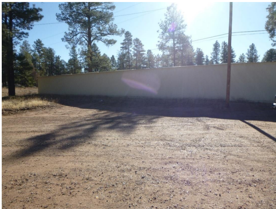
Figure C.65. Backside of Garage 12 Bays (13-91), view east.
