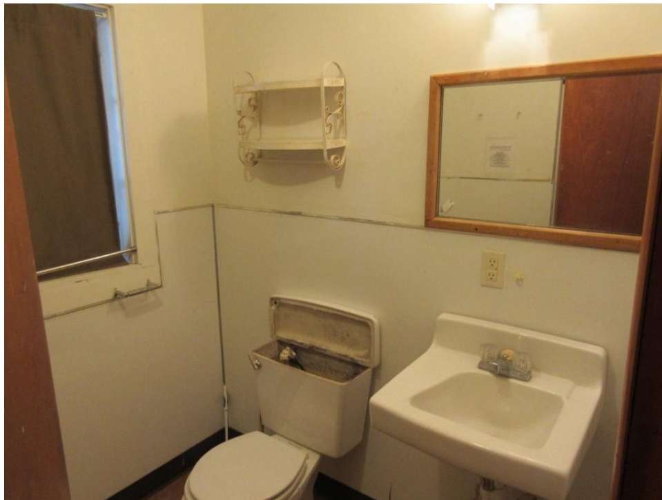
Figure C.22. Bathroom example in Engine Quarters (11-60), view from door.
