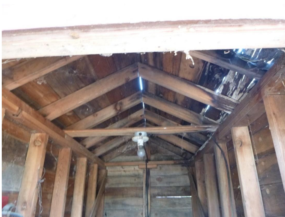
Figure C.48. Wooden structure of Old Well House (16-71).
