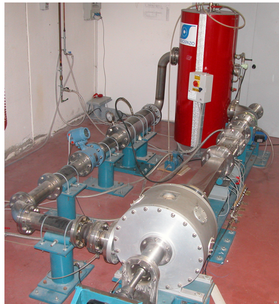
Figure 1. The Cavitating Pump Rotordynamic Test Facility (CPRTF).
