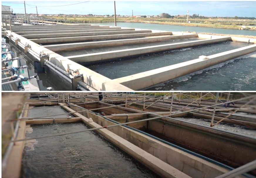
Figure 20. Production tanks (up to 20 m 2 ) @Inês Oliveira
