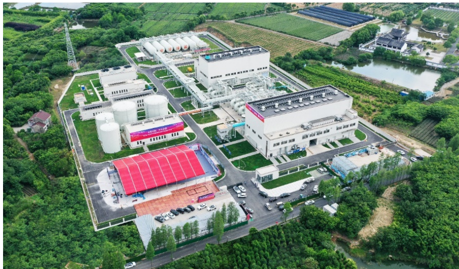
Fig. 1 Aerial panorama of Jintan Salt-cavern Compressed Air Energy Storage National Demonstration Project.
