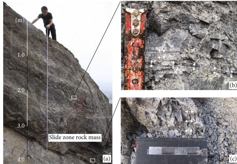
FIGURE 21: Fragmentation of the bedding fault rock mass. (a) Trench, (b) close-up view of the rock mass shows tension cracks, and (c) rock mass dilatation due to earthquake induced tension fracture.
