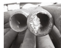
FIGURE 4: Scale blockage in the wellbore.
