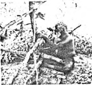
9. Side rails are lashed to the posts with bush string and vines ( vigna marina ).
