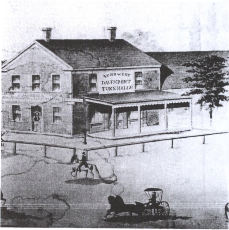
Northwest Turner Hall, Davenport, Iowa, 1871.
