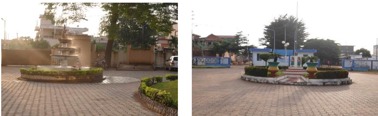
Figure 8. Driveways at public service buildings with permeable pavements, Cotonou 2014.
