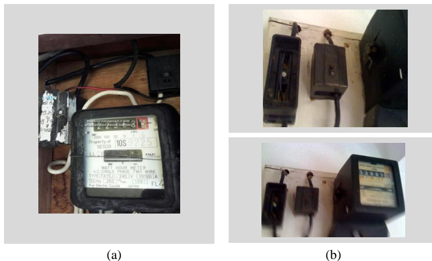
Figure 1. Illegal connection via (a) direct connection to main supply [5] and (b) bypass wire [6]
