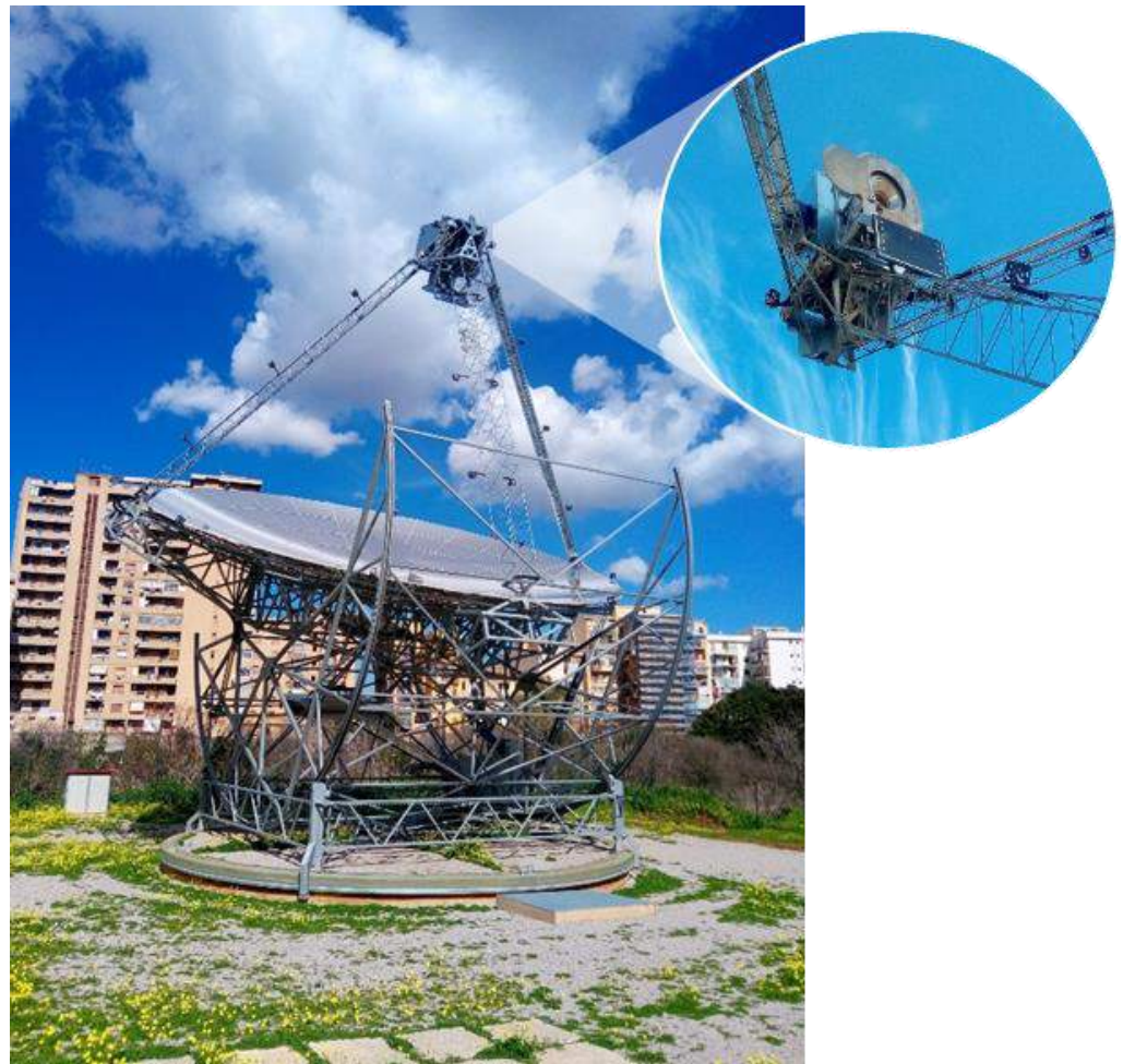
Figure 1. The dish–Stirling concentrator plant that is installed at the University of Palermo.
