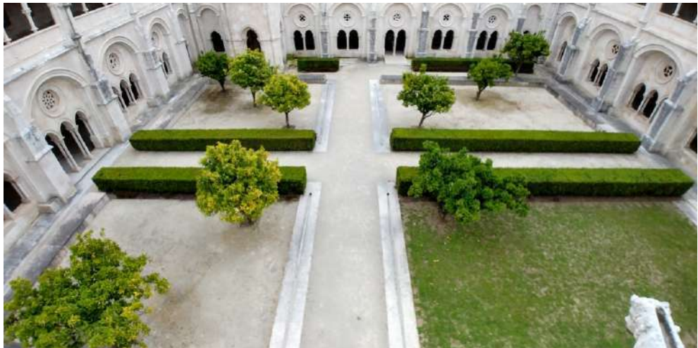
Fig. 6 - Alcobaca Monastery cloister – recovery project by G. Byrne (image of Dessi, 2015-18)
