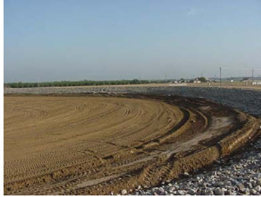
Figure 7. Earthwork to establish reservoir levees and rip rap for levee protection.
