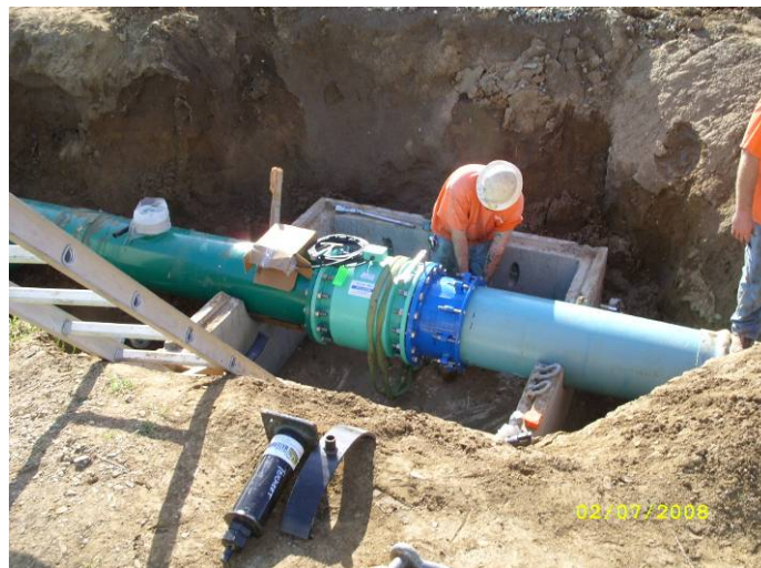
Figure 11. 1N pump station magnetic flow meter
