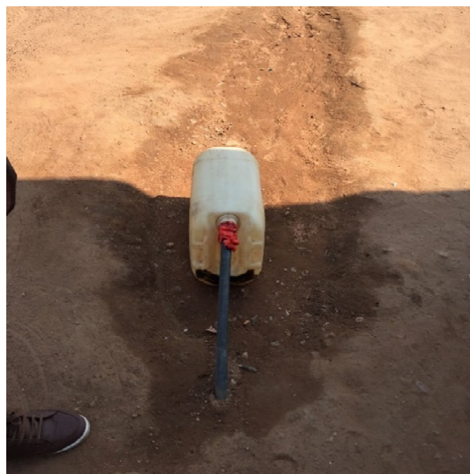
Figure 4. A pipe coming out from the ground that sporadically has water running out from it in Mopani.
