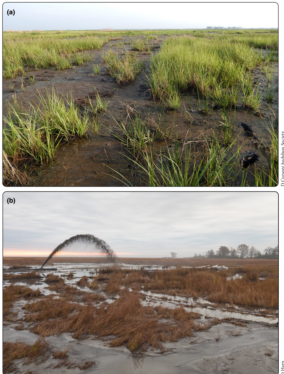
Figure 4. (a) Passive revegetation following (b) thin-layer placement at Blackwater National Wildlife Refuge.
