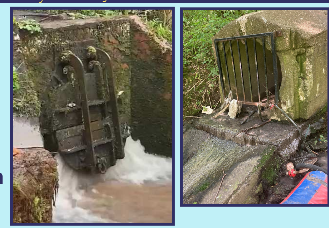
Figures 1 & 2. Combined sewer overflow outlets at two sample sites in Sheffield.
