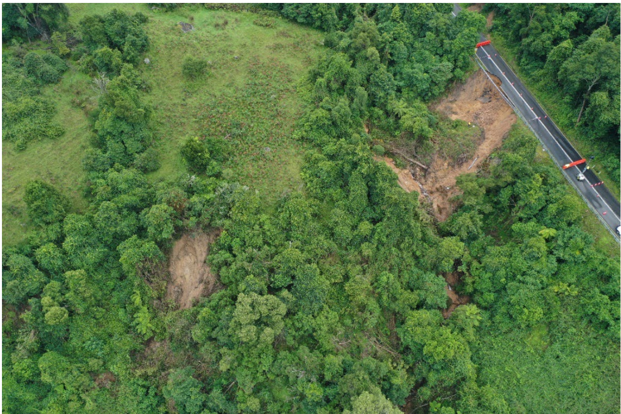
Figure 12. Barrengarry Mountain Road showing the extended flow component of the landslide and an adjacent debris flow.
