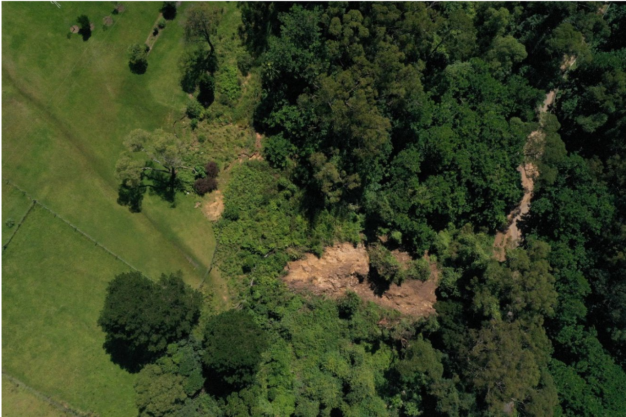
Figure 26. RPA photograph of debris flow above Harry Graham Drive. RPA photo by Flentje 10 th March 2022.
