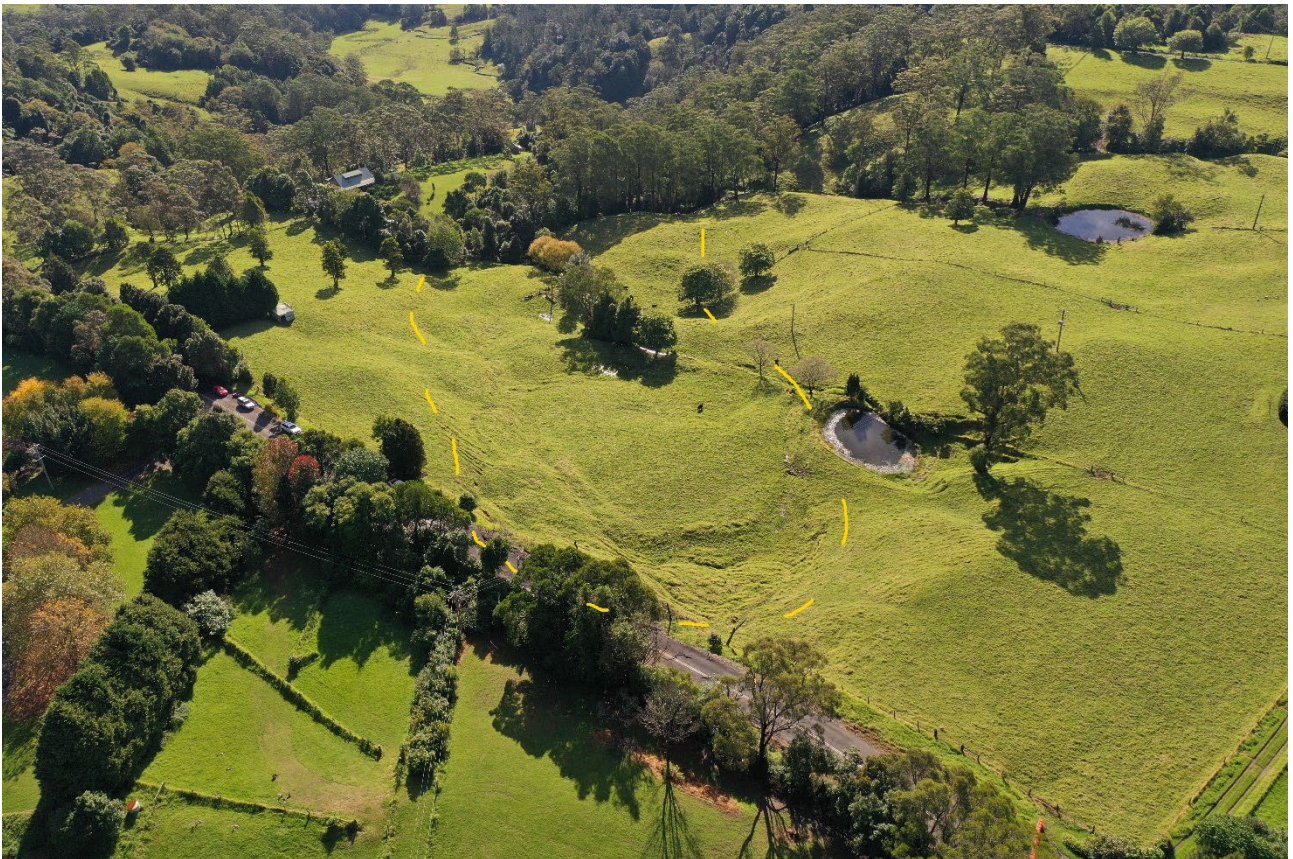
Figure 32. RPA oblique photograph of Wattamolla Road. Approximate landslide boundary outlined in yellow. Photo by Flentje 26 th April 2022.
