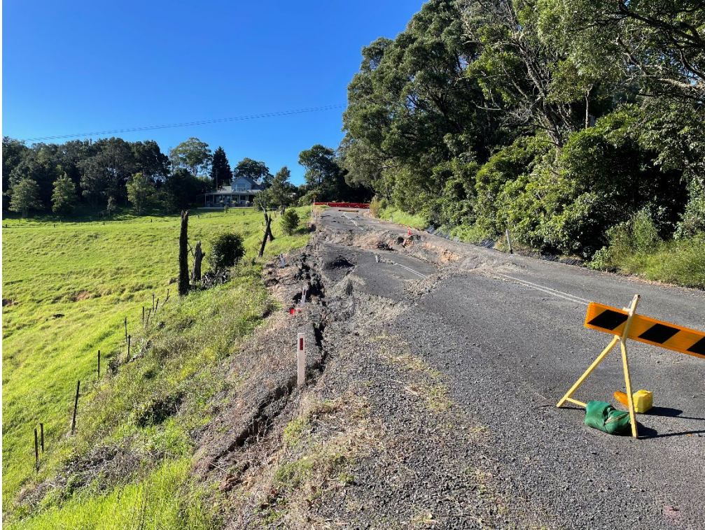
Figure 31. Major slide which closed Wattamolla Rd on March 2. Photo by Larkin 19 th May 2022.
