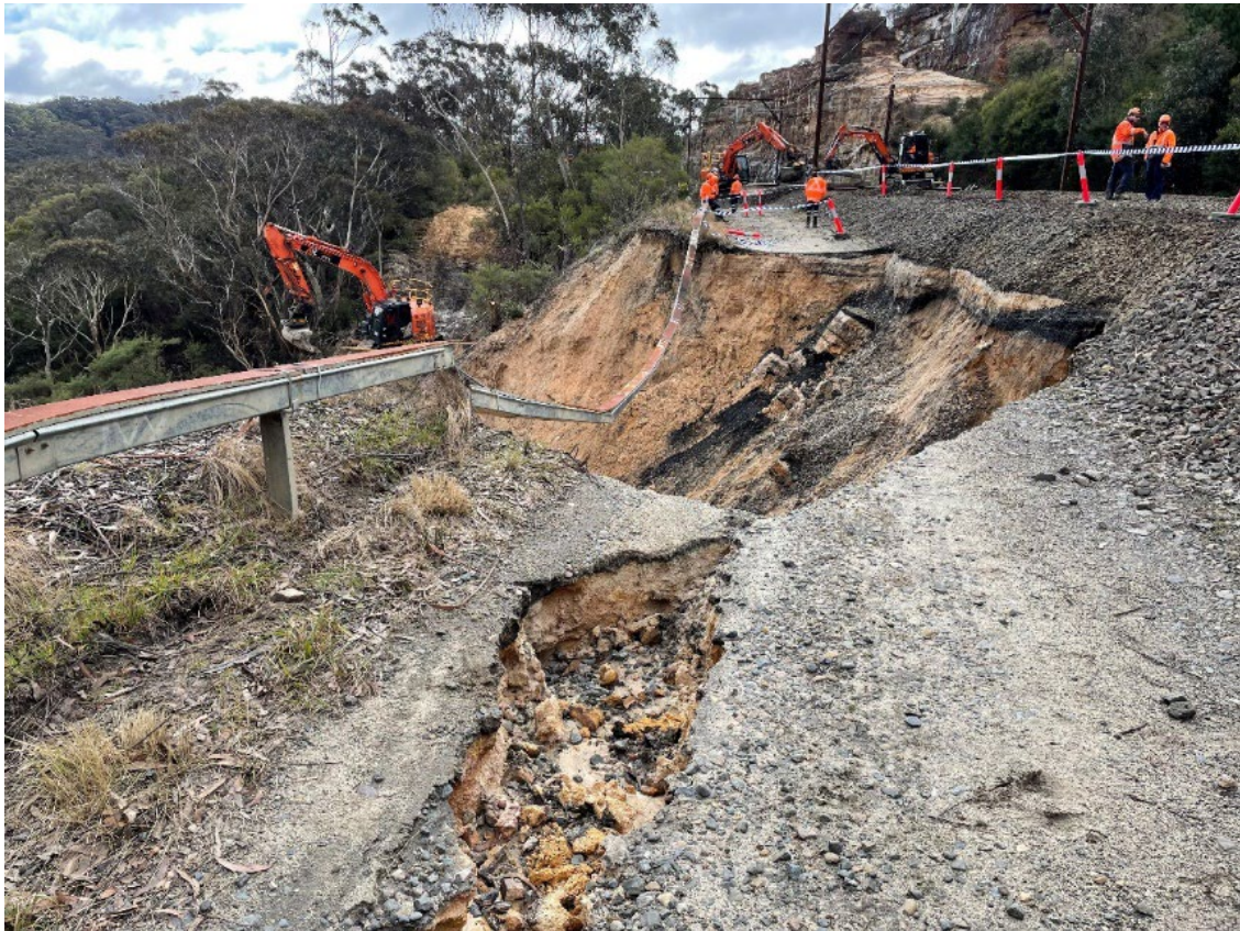
Figure 22. Major slide which closed Main West at Blackheath around 11pm July 4. Photo by Larkin 8 July 2022.
