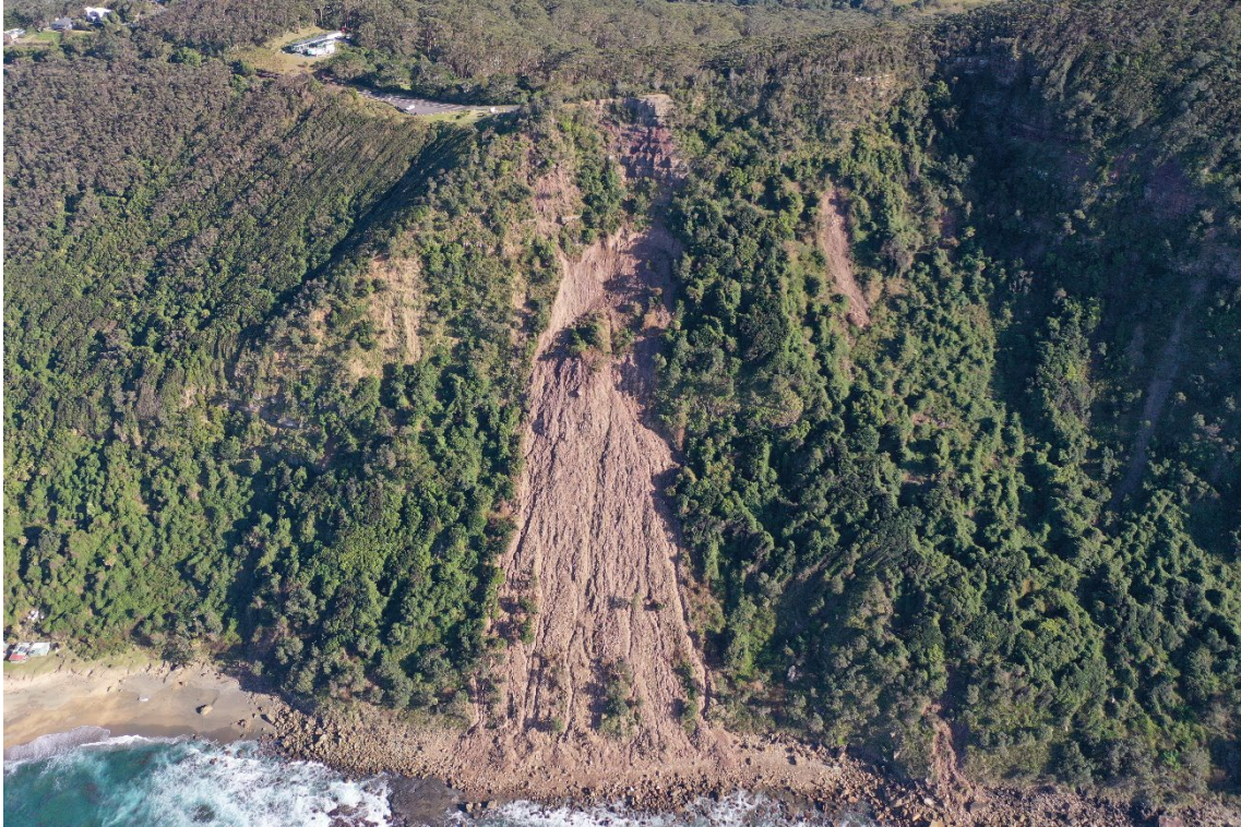
Figure 30. Bald Hill Claystone and Bulgo Sandstone cliff face below Otford lookout at the south end of the Royal National Park. RPA photo by Flentje 8 th August 2022.
