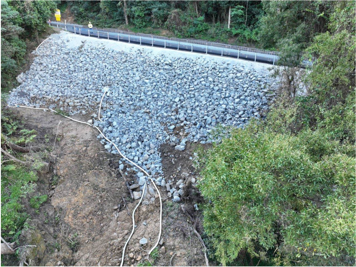
Figure 13. Barrengarry Mountain Road rockfill. RPA photograph by Horan, late July 2022.
