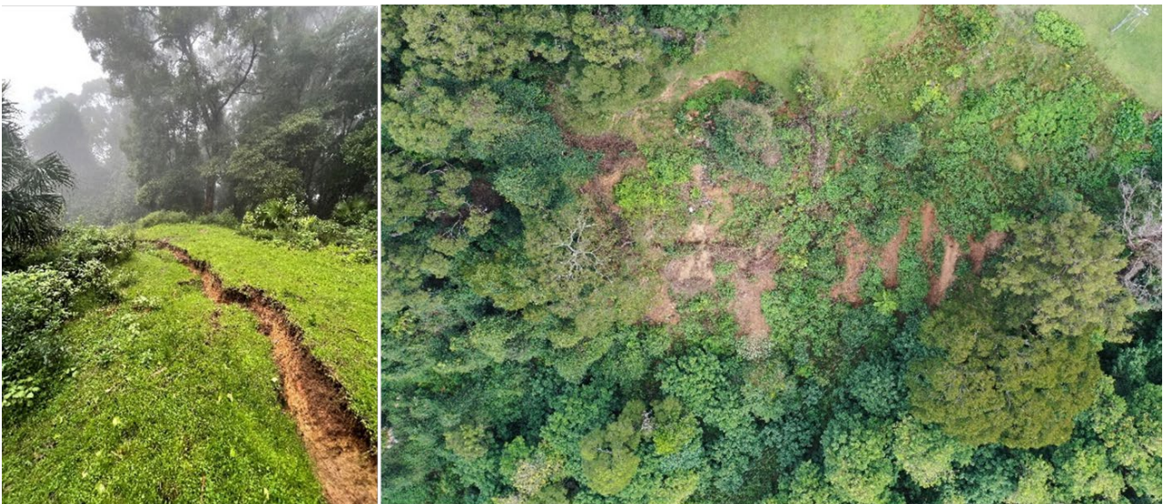
Figure 6. At the eastern edge of the Stanwell Park Claystone Terrace, the colluvium breaks away and slides over steepening slopes. This crack was reported by the owner and mapped on the 7 th March at up to 600mm, with a backscarp at ~75°. After 4 weeks this scarp had grown to over 2m in several locations and was observed on the ground and by RPA on the 5 th May. The toe of this slide had by then flowed over the Scarborough Sandstone cliff face as a number of debris flows, stopping short of MOR. (RPA photo by Flentje).
