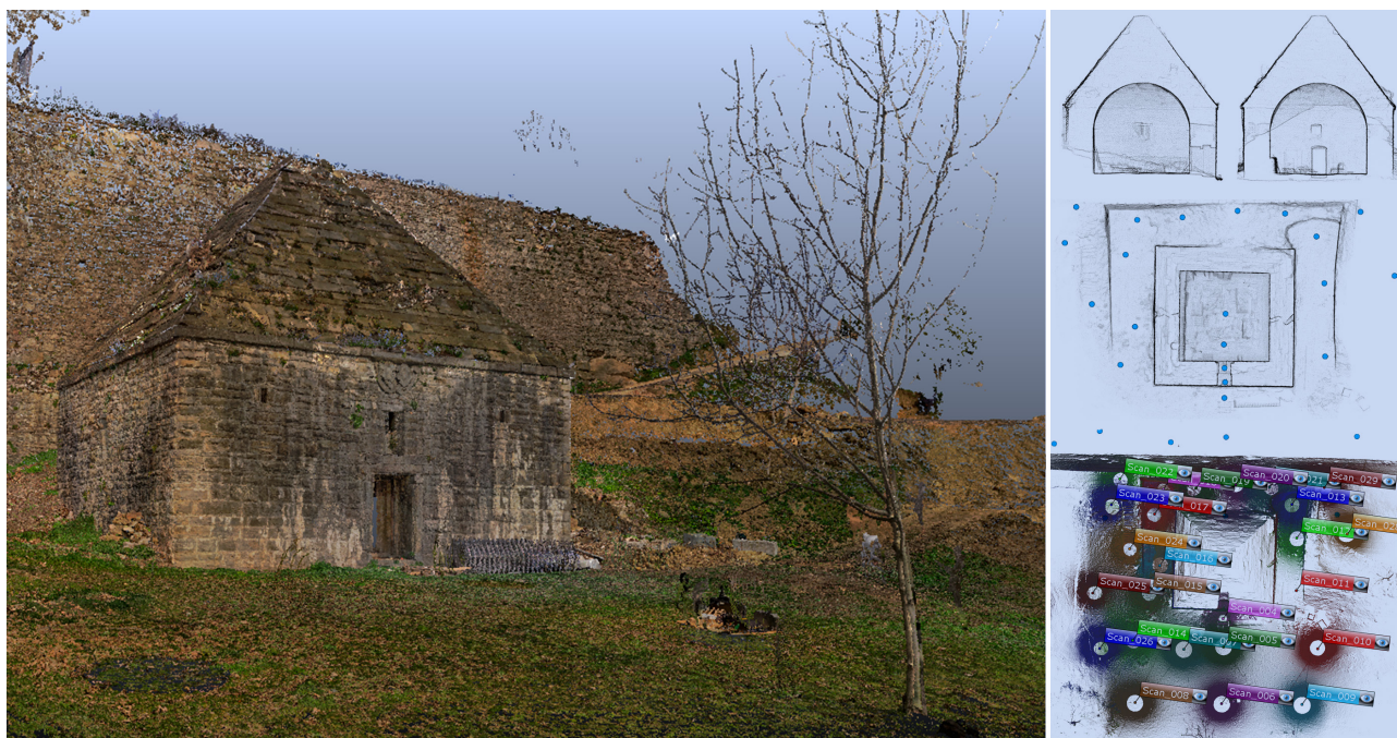
Figure 3. 3D laser scanning: point cloud model and data elaboration
