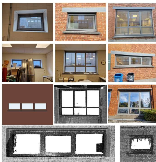
Figure 4: Selection of used images. Containing RGB images of the real life objects, renders of the BIM model and Point cloud.
