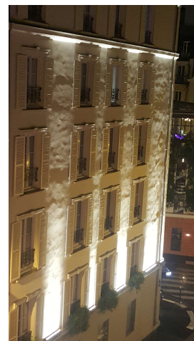
Figure 1. The planarity defects of the facade are highlighted by a grazing lighting, which is the basic principle of RTI.
