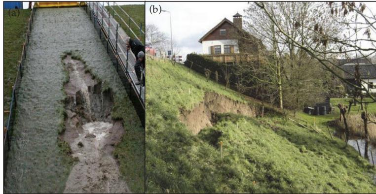
**Figure 1.** (a) Dike cover erosion on the landward slope and toe during wave overtopping field tests in the Netherlands (Photo by Juan Pablo Aguilar Lopez). (b) A slope instability of a grass-covered clay dike in the Netherlands [17].
