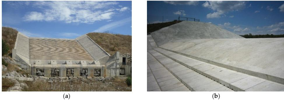
**Figure 1.** (a) The Barriga dam (Burgos, Spain). (b) The upper area detail of the WSB chute spillway of the Barriga dam.
