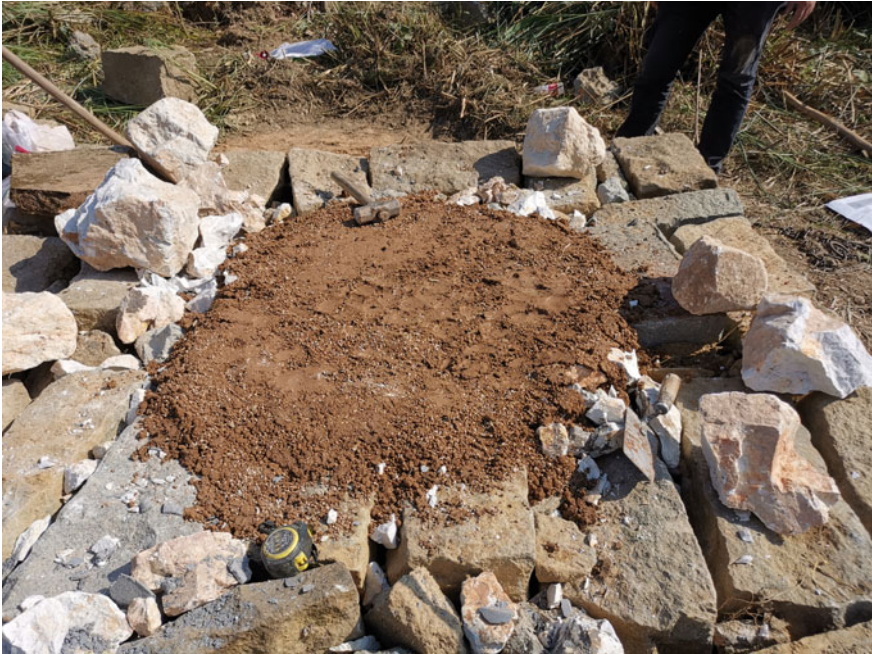
Fig. 7.7 The foundation of the furnace is crucial. The soil underneath the designated area for the furnace was tamped
