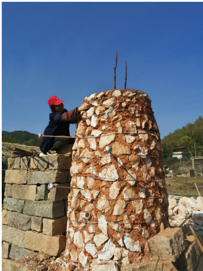
Fig. 7.17 Fill the gaps between quartz with red clay
