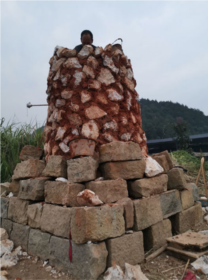
Fig. 7.16 Install a thermometer during the construction of the furnace
