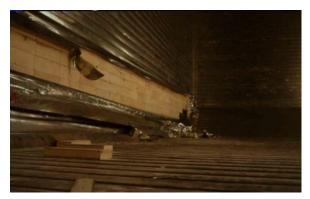
Figure 1-5: Failure of the primary barrier due to sloshing [22]
