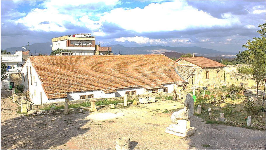
Fig. 9 North façade view of the Sidi Ghanem Mosque
