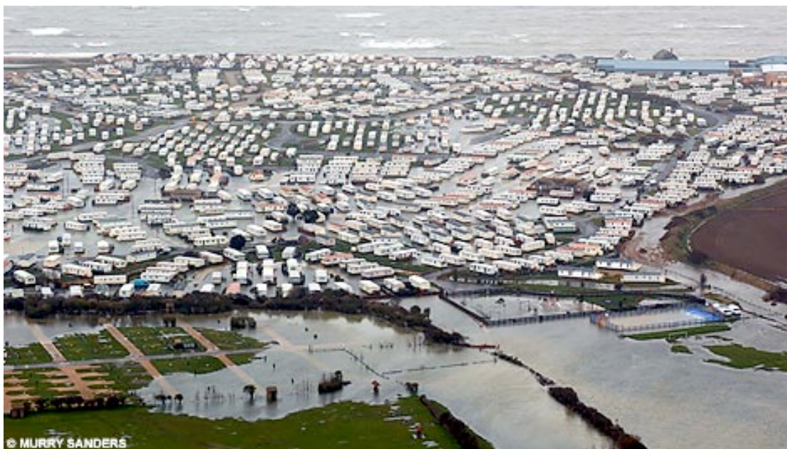
Figure 3.2: Flooding to a caravan site at Medmerry, on the Manhood Peninsula, in during the 10 th March 2008 storm surge (looking southwards) caused by a breach in shingle barrier beach defences (source: Daily Mail, 2008).
