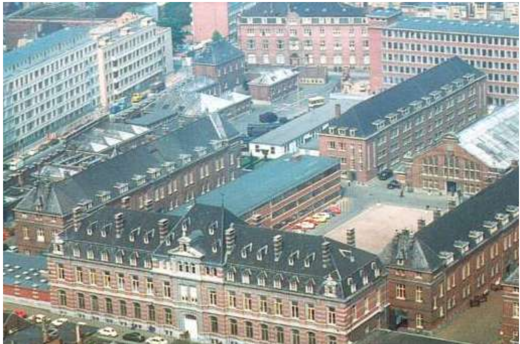
Aerial view of the former Ixelles barracks undergoing rehabilitation
