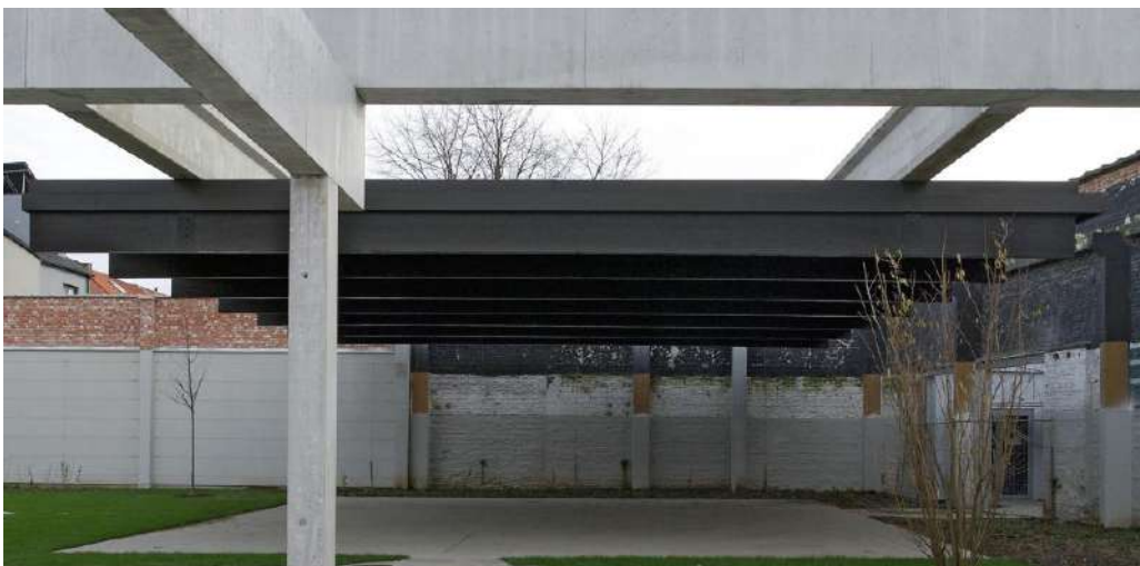
From top to bottom: (1) Original situation. (2) Storage of the beams on site after dismantling. (3) Reuse in the new project.
