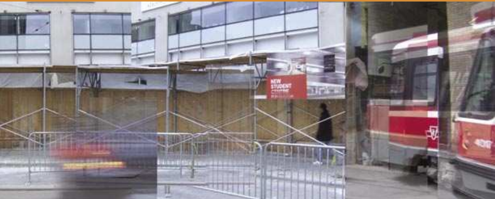
ABOVE WORK IN PROGRESS: OCAD CONSTRUCTION ON McCAUL STREET
