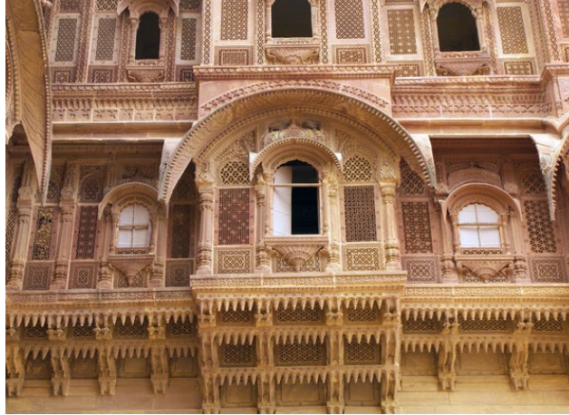
Figure 26: Jali Work at Patwon Ki Haveli, Rajasthan, India
