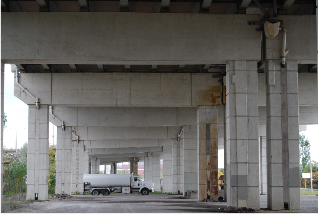
FIGURE 3.2: Highway overpass location
