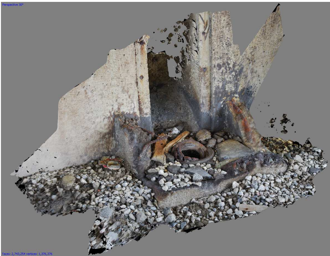
FIGURE 4.1: Raw photogrammetry scan of highway detail
