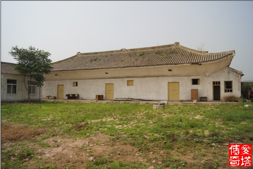
Figure 14 Main hall of the Tangwang temple. Cap and block are wrapped in a layer of white lime, source: http://blog.sina.com.cn/s/blog_4a877d4d0102erzw.html
