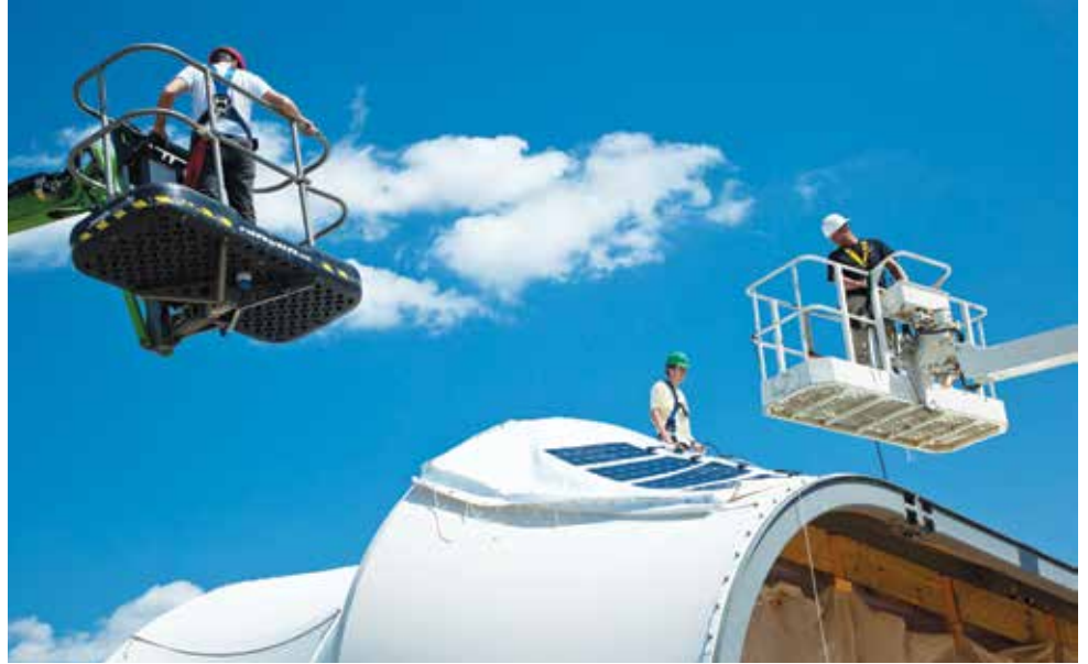
Sheets of flexible photovoltaic cells replace stiff solar panels on the curvy roofline. And thanks to photoluminescent paint on the interior, there's no need to turn on a light to use the bathroom at night.
