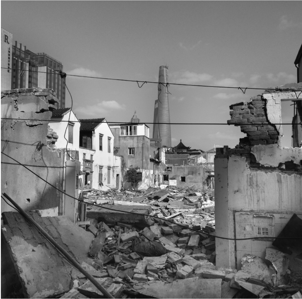
37. HUTONG DEMOLITION. SHANGHAI, CHINA. 2014
