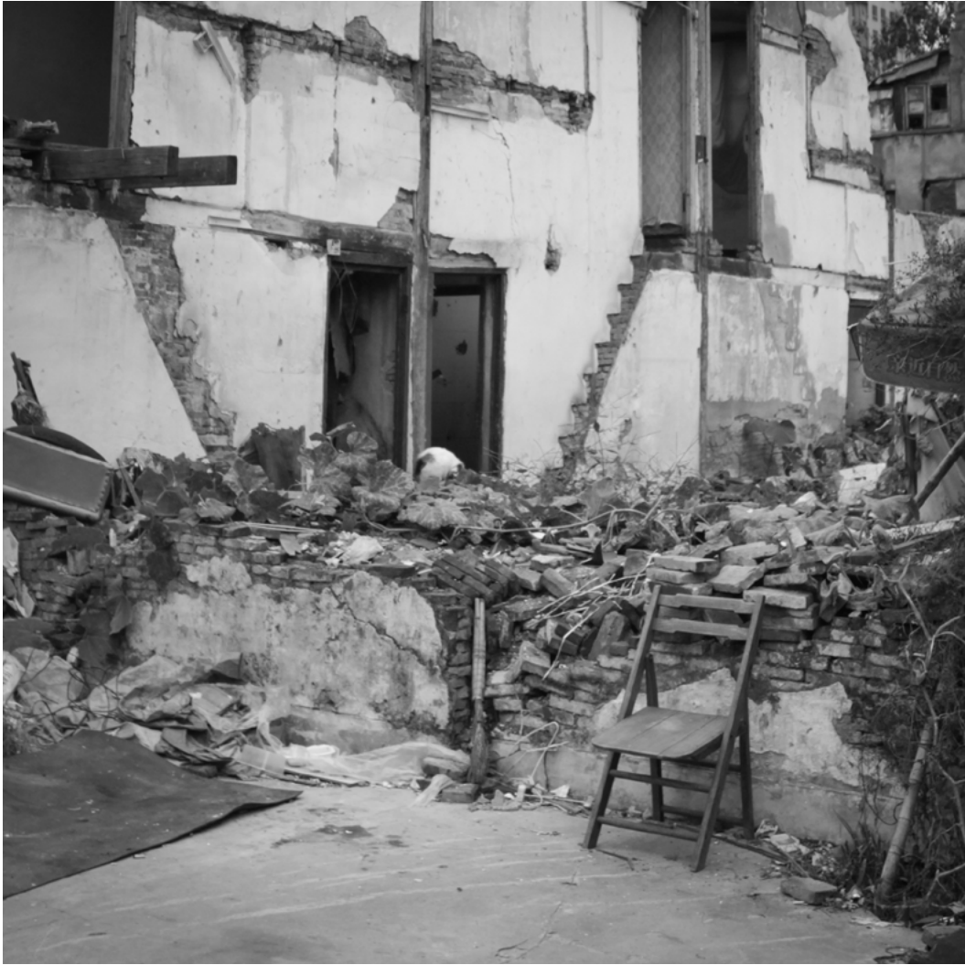
23. HUTONG DEMOLITION. SHANGHAI, CHINA. 2014
