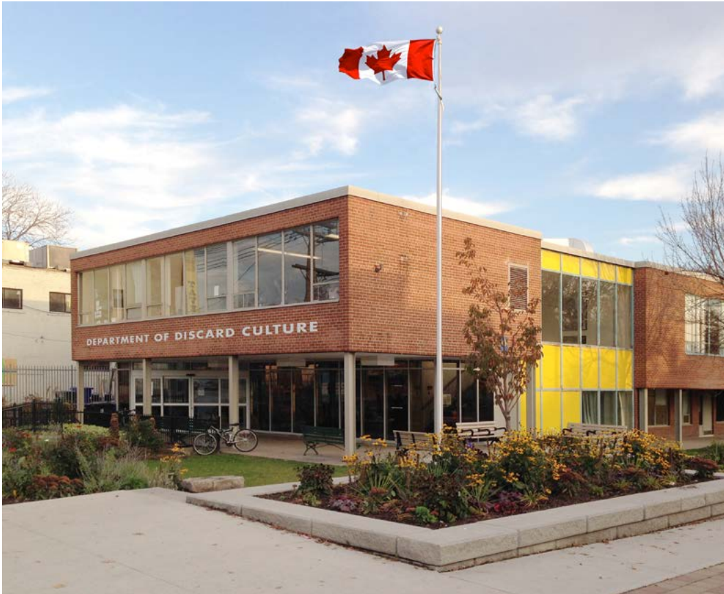
2. DEPARTMENT OF DISCARD CULTURE, BUILDING (FRONT VIEW), 2015
