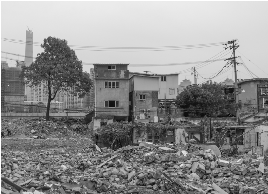
22. HUTONG DEMOLITION. SHANGHAI, CHINA. 2014
