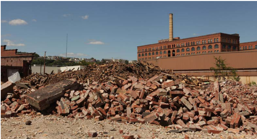
38. FACTORY DEMOLITION. PITTSBURG, PA. 2014
