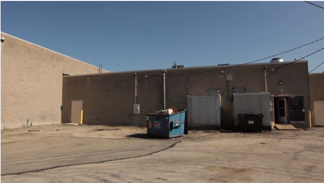
18. DUMPSTER. PITTSBURG, PA. 2014
