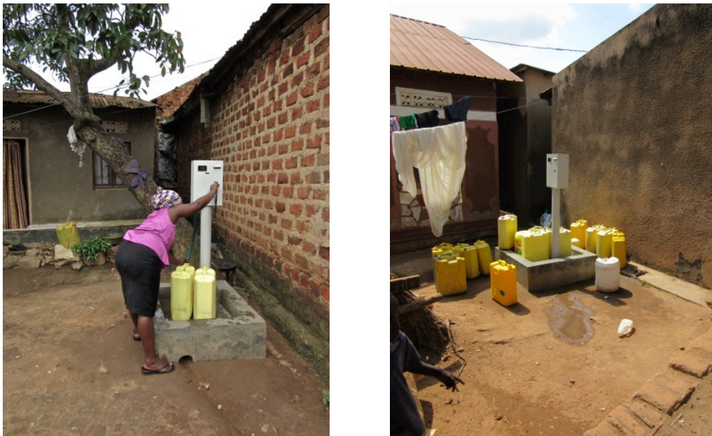
Figure 27 Prepaid water standpipes in use
