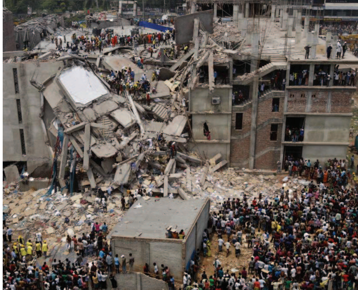
Fig. 10 | Rana Plaza Collapse, Dhaka, Bangladesh (Source: Rijans - https://www.flickr.com/photos/rijans/8731789941/ )
