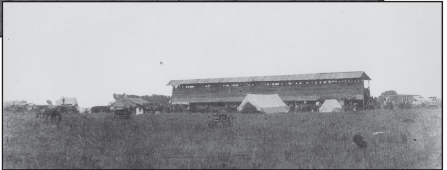
Top: Grandstand at the horse track under construction (OHS Research Division).
