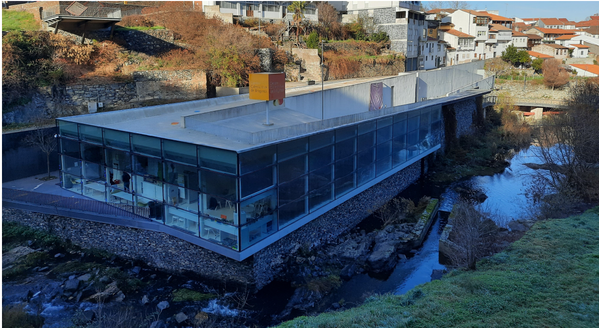
Figure 3.1: The CCVB on the bank of the Fervença River.
