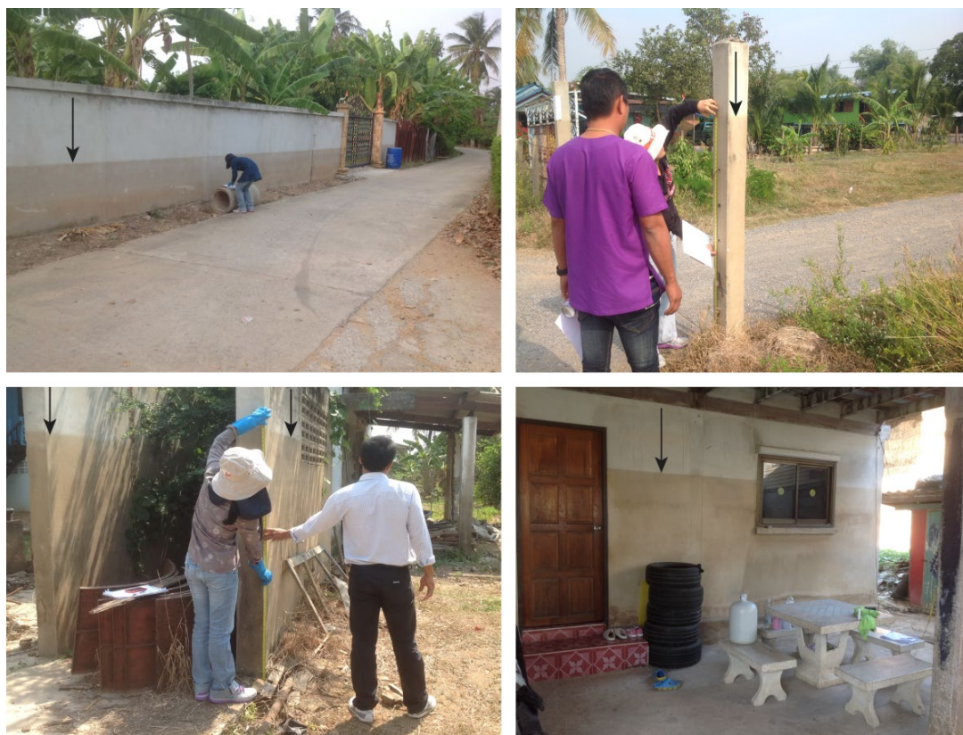
Figure 2 The examples of the traces of flood levels on the concrete poles (top right), the temple wall (top left) and the buildings (bottom) located in the Chao Phraya River Basin.
