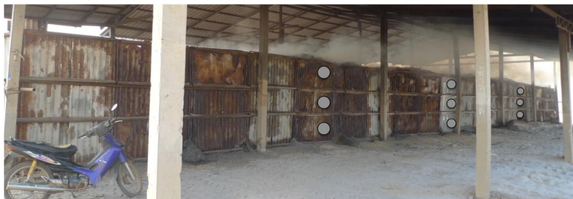
● The monitoring point of the temperature
